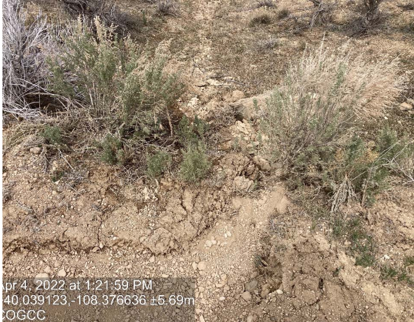
Lack of stabilization/compaction/erosion
