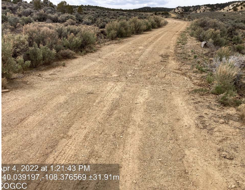
Lack of stabilization/compaction/erosion
