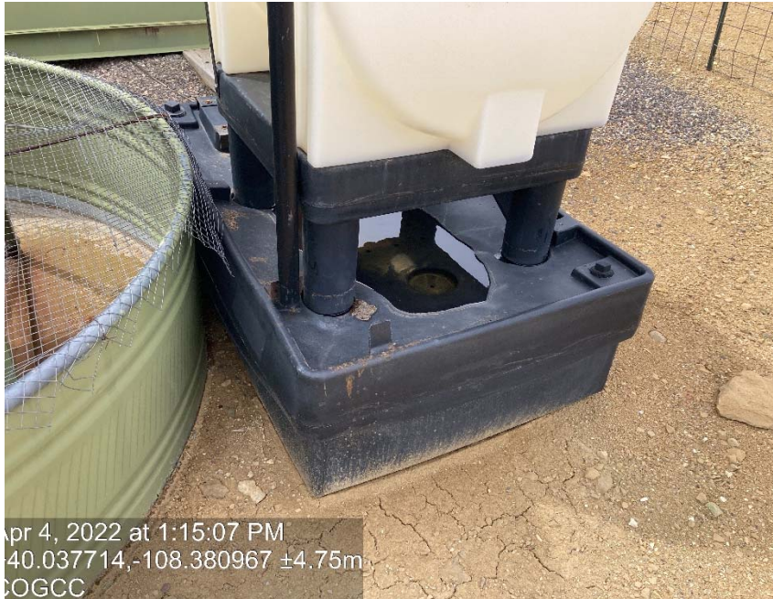
Chemical tank containment full of fluid
