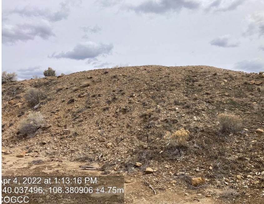
Lack of stabilization/compaction/erosion
