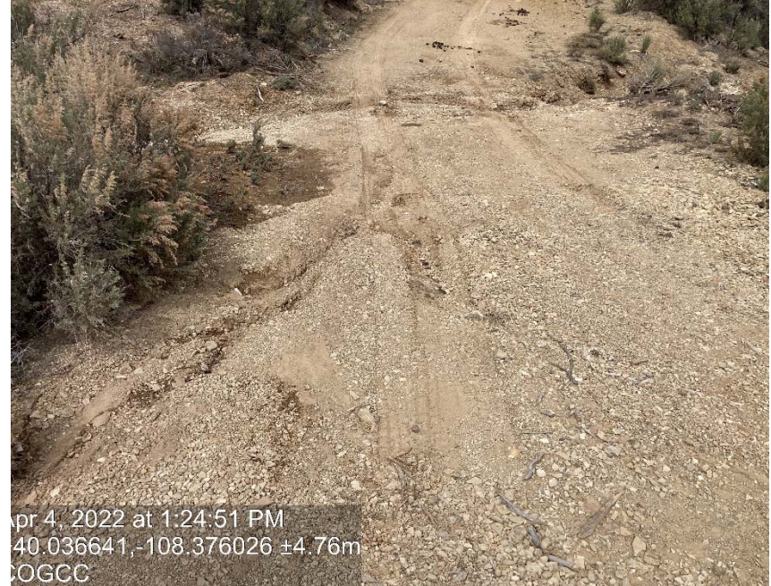
Lack of stabilization/compaction/erosion
