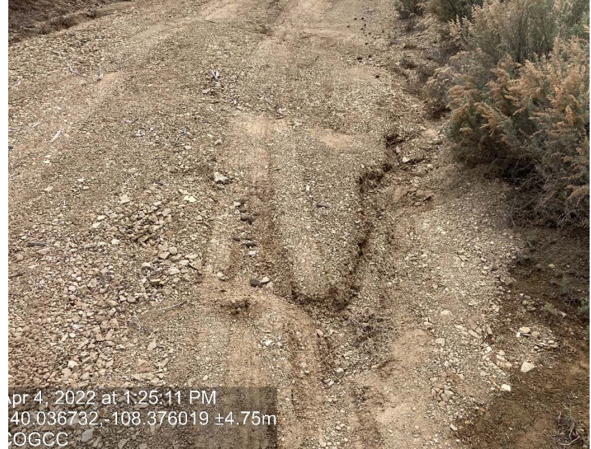
Lack of stabilization/compaction/erosion
