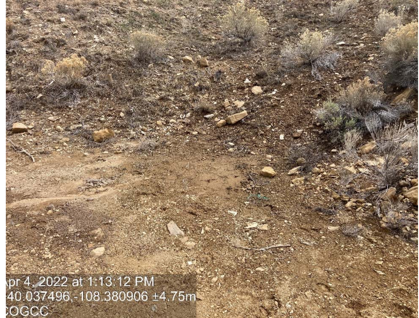
Lack of stabilization/compaction/erosion
