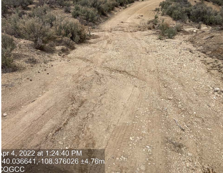
Lack of stabilization/compaction/erosion
