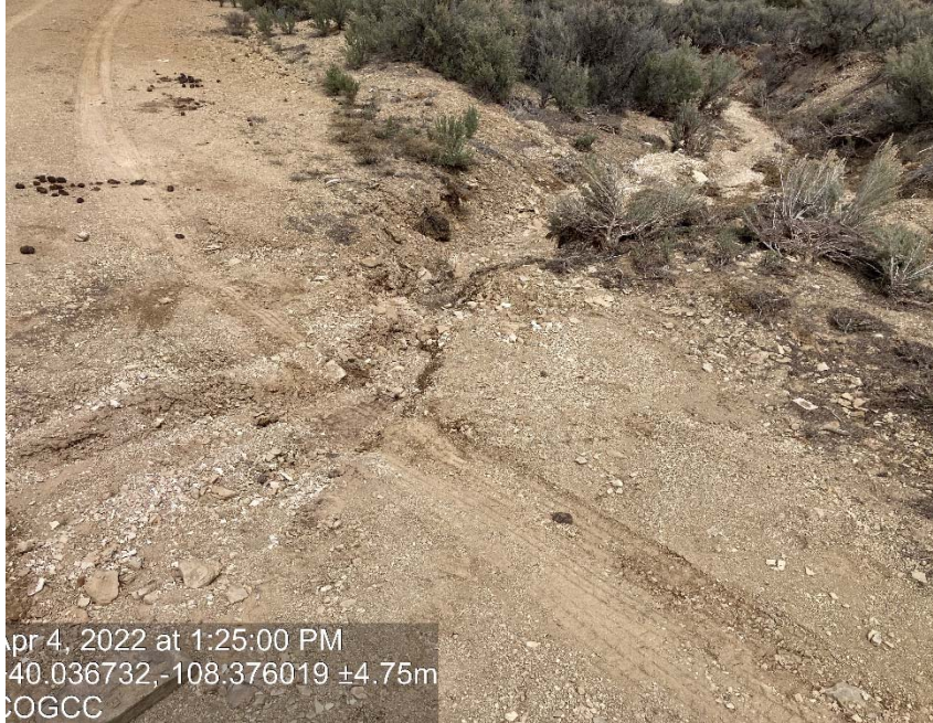
Lack of stabilization/compaction/erosion
