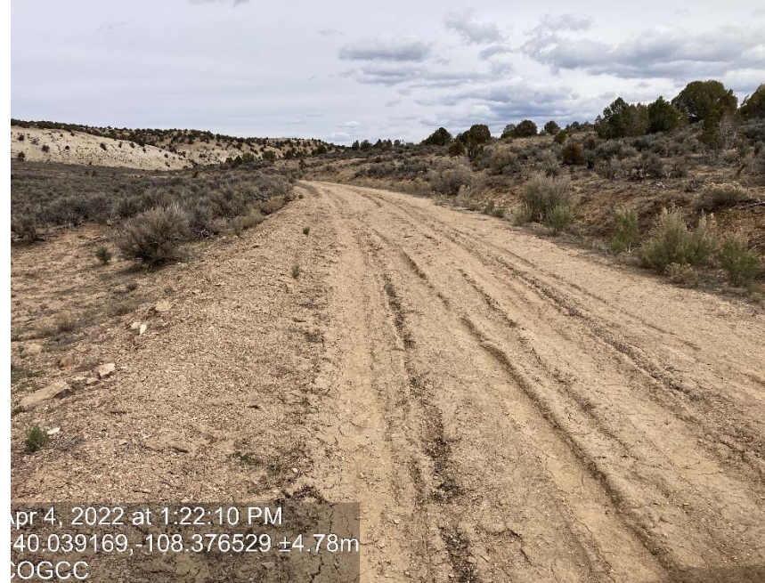
Lack of stabilization/compaction
