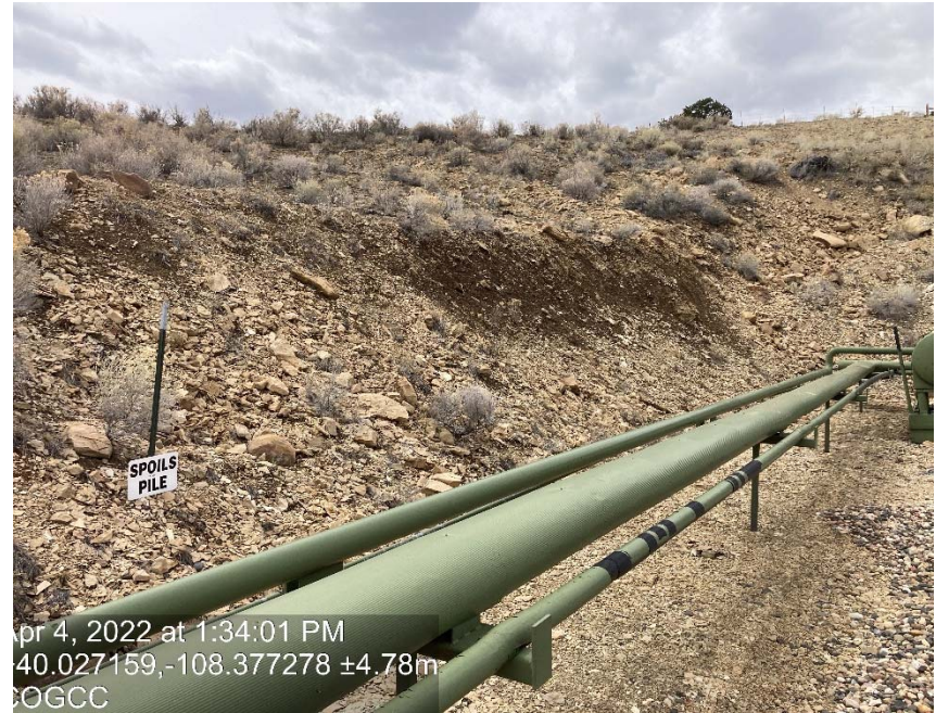
Lack of stabilization/compaction/ erosion
