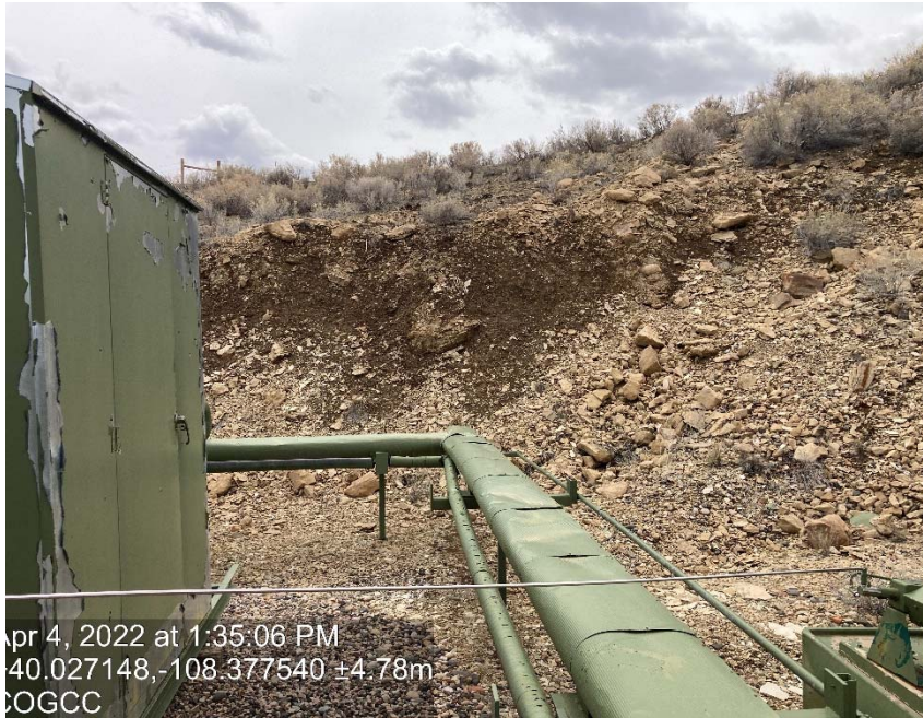
Lack of stabilization/compaction/ erosion
