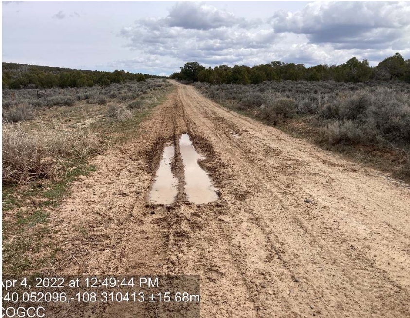
Lack of stabilization/compaction
