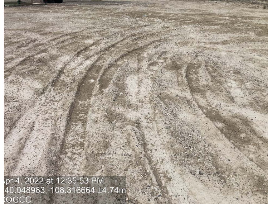
Lack of stabilization/compaction
