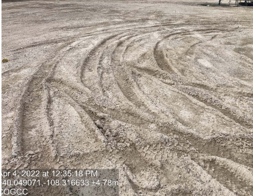
Lack of stabilization/compaction
