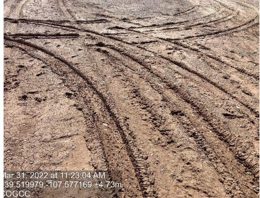
Lack of stabilization/compaction
