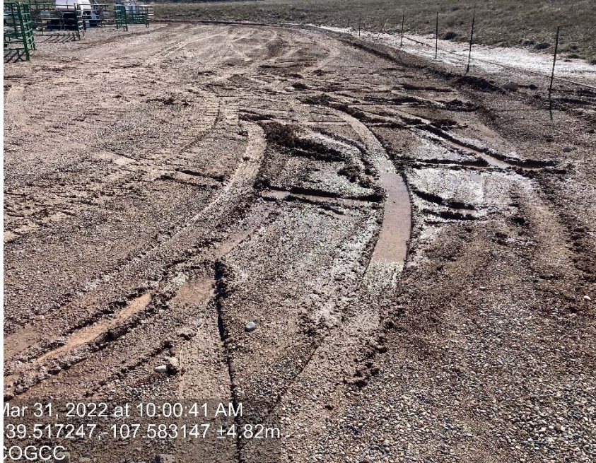
Lack of stabilization/compaction
