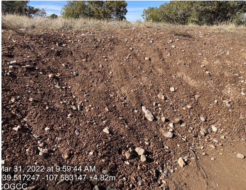
Lack of stabilization/compaction/erosion
