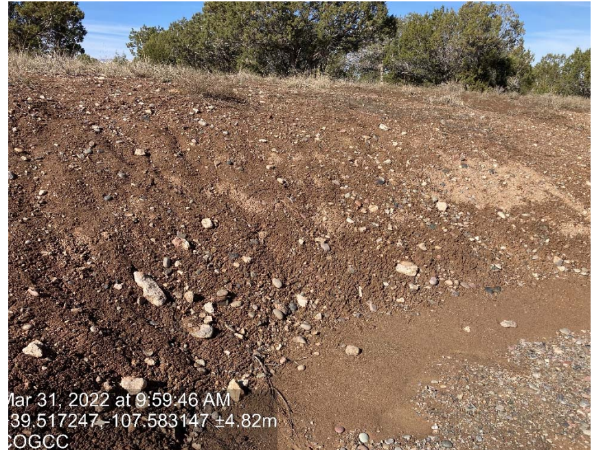
Lack of stabilization/compaction/erosion
