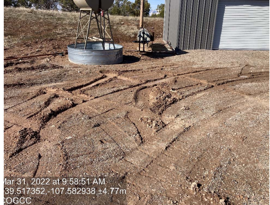
Lack of stabilization/compaction
