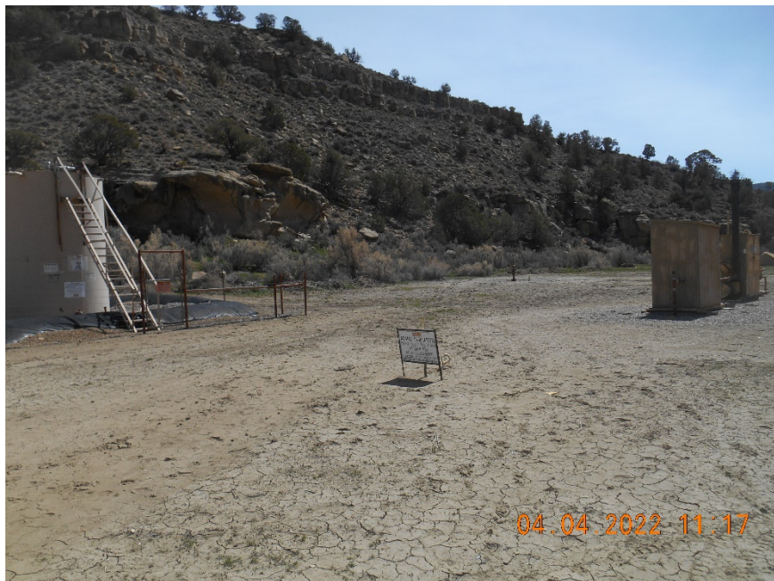
Location overview looking SE.
