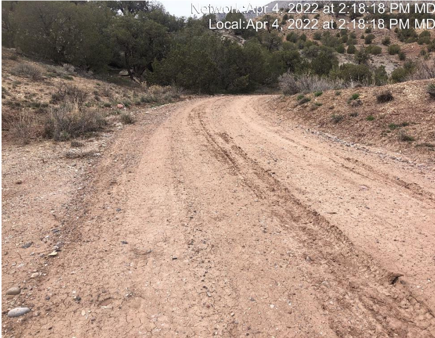
Photo #6357 Insufficient tracking BMP at entrance to location.
