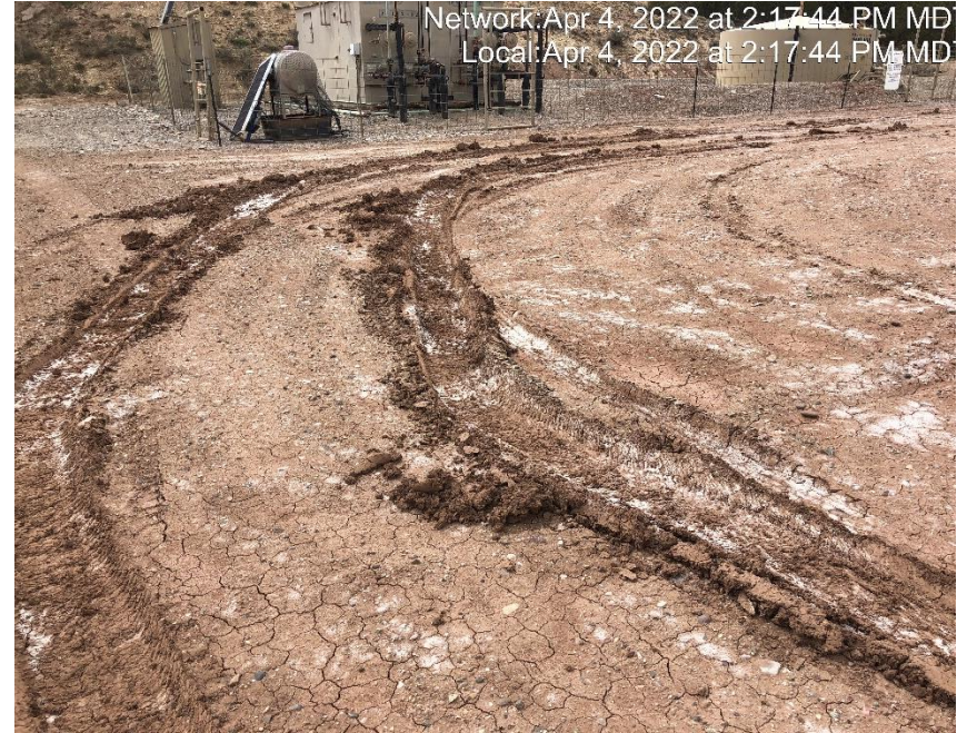
Photo #6356 Location lacks stabilization.
