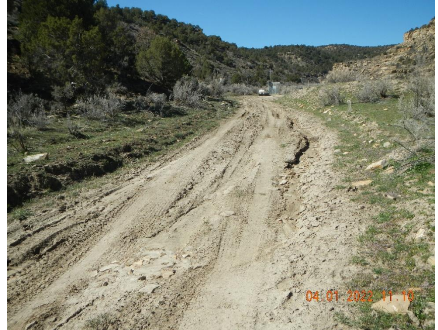
Rill and lack of stability of roadway.
