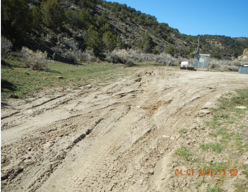
Rill wash off location onto roadway.
