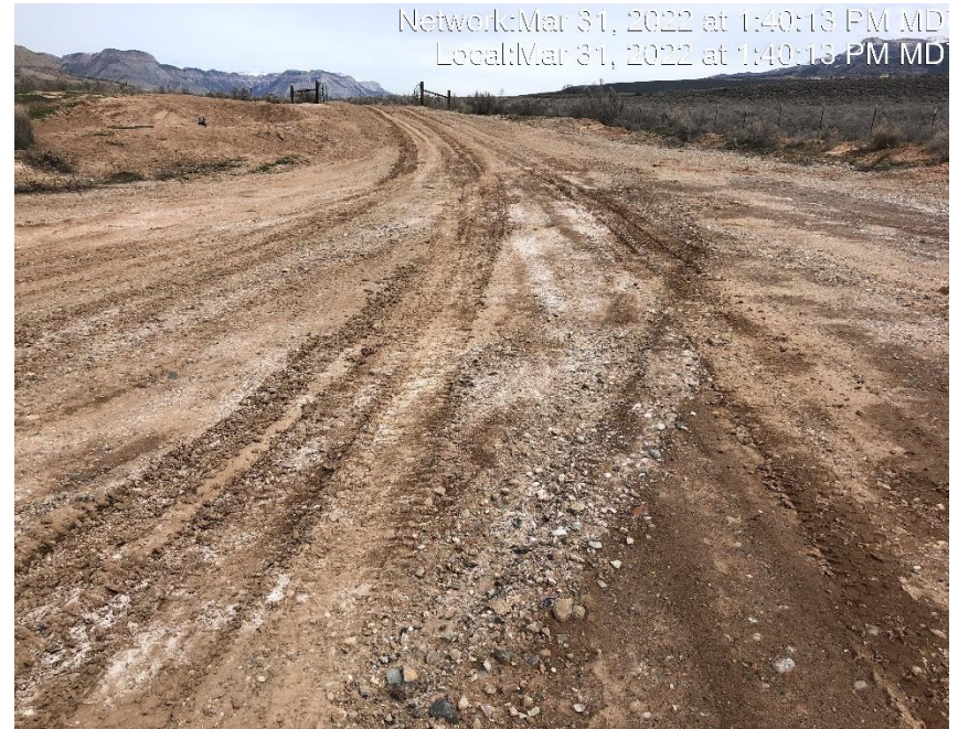
Photo #6338 Insufficient tracking control located at entrance to location.
