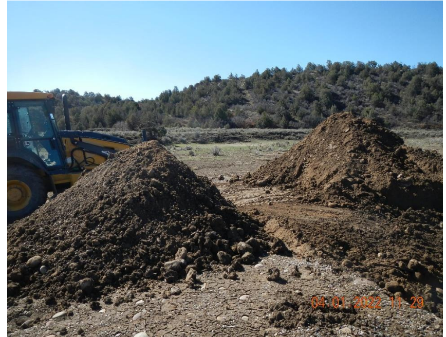
Stockpiled material next to excavation. Material in the foreground is freshly excavated, backfill material in background.
