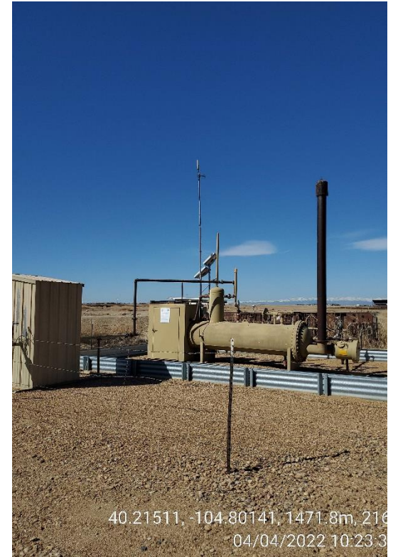
Photo 3 Production Separator
