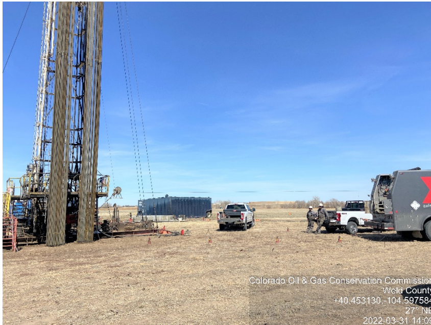
Photo #1 Francen 19-30 (05-123-21984) Wellsite Plugged & Abandoned | PA Plugging Operations: Cementing Set CIBP, cement
