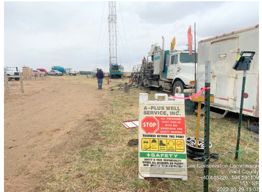
Photo #2 Printz 2-31 Wellsite Plugged & Abandoned | PA Plugging Operations: Kill well | WK Site safety signage prior photo
