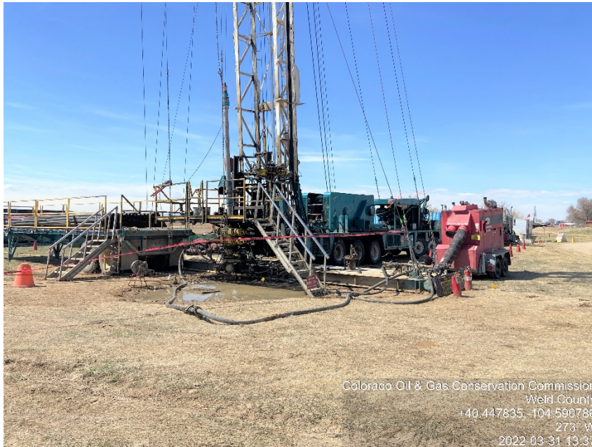
Photo #1 Printz 2-31 (05-123-13199) Wellsite Plugged & Abandoned | PA Plugging Operations: Cementing Courtesy plug, cement to surface
