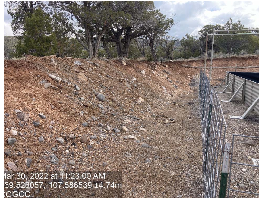
Lack of stabilization/erosion
