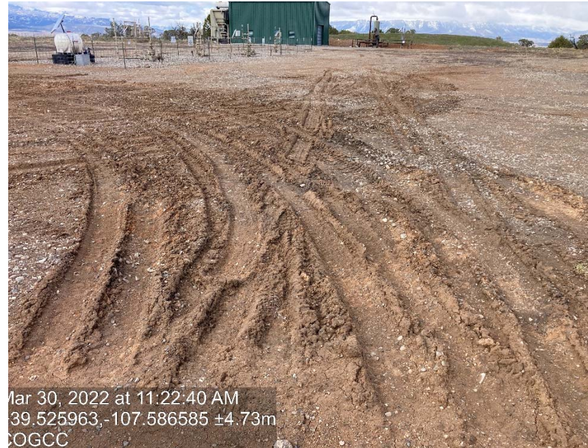
Lack of stabilization/compaction
