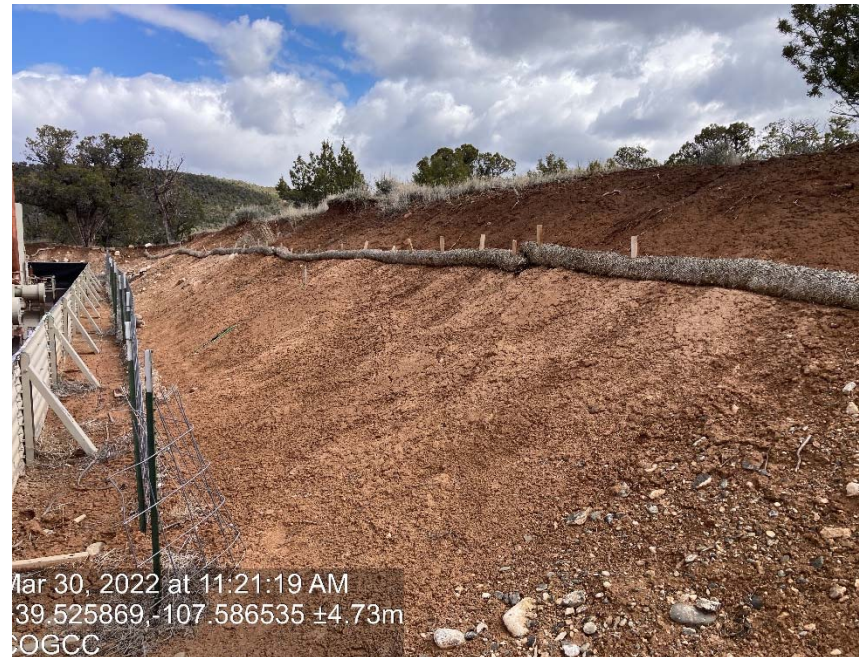
Lack of stabilization/erosion. BMP's are failing
