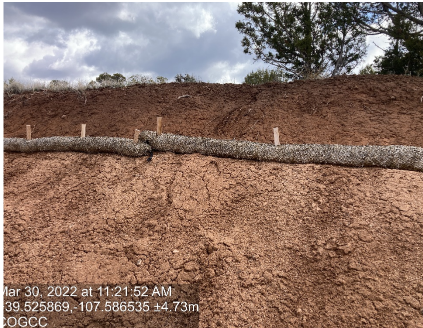
Lack of stabilization/erosion. BMP's are failing
