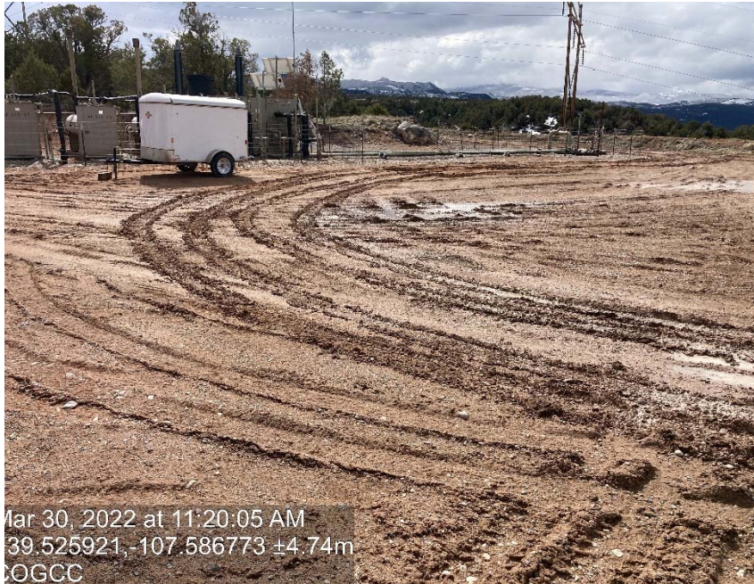
Lack of stabilization/compaction
