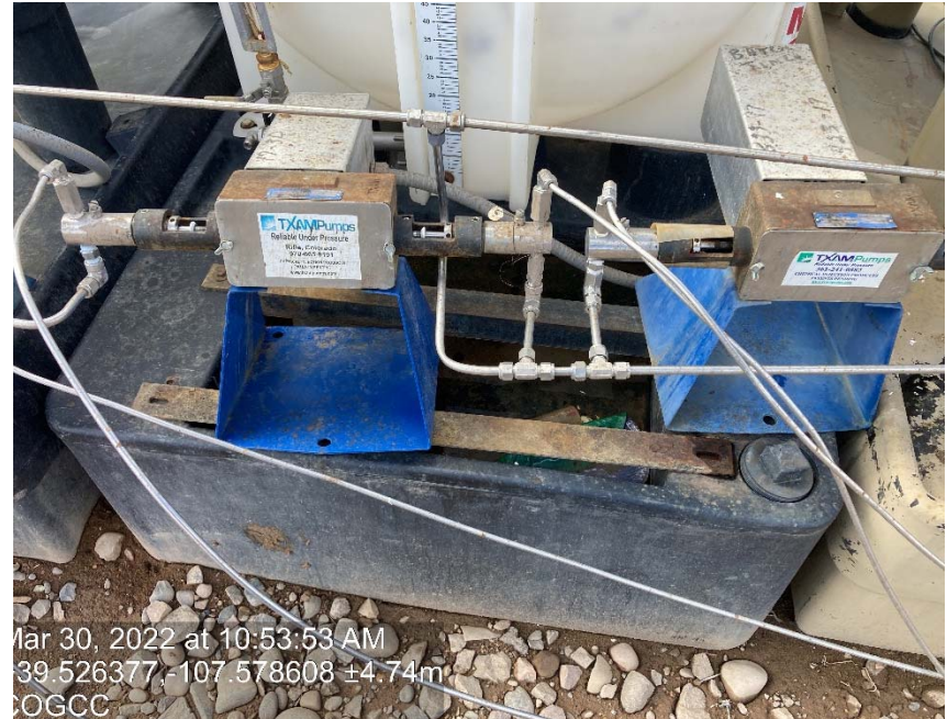
Chemical tank containment full of fluid
