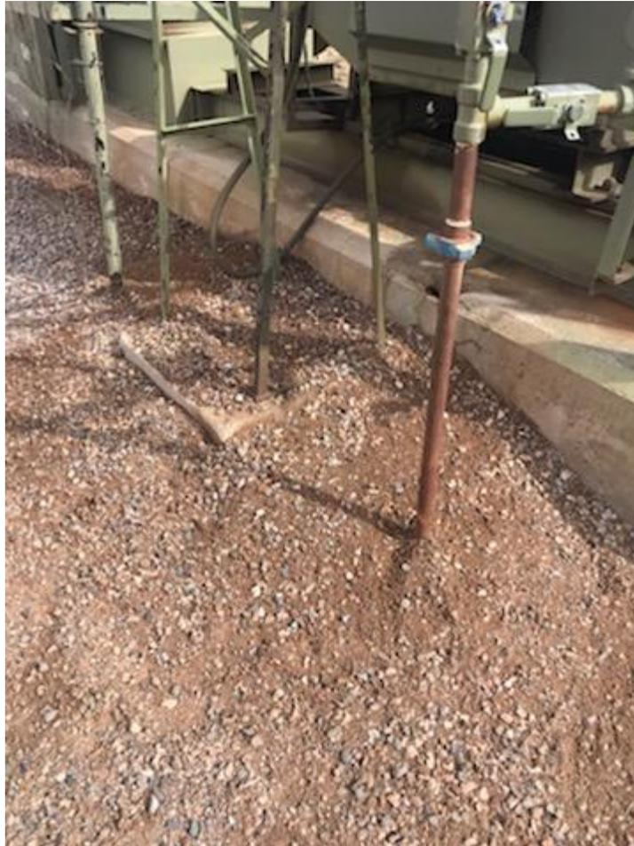
**Comment:** The concrete pad and soil beneath the prime mover are wet and stained.
