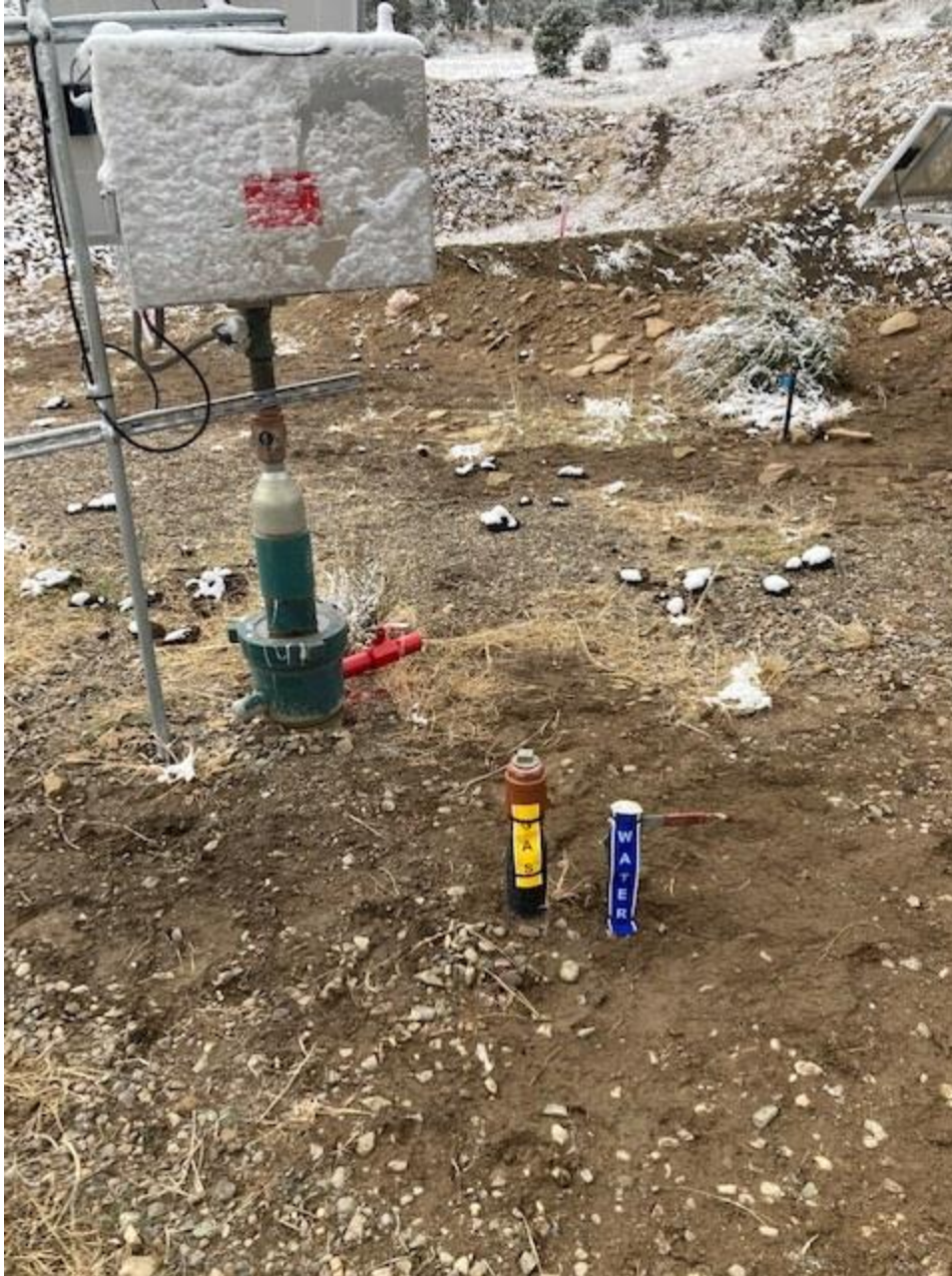
Removed part of unused equipment and properly marked to comply with Rule 606
