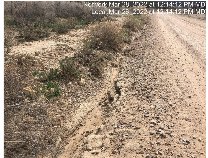
Photo #6317 Insufficient velocity checks in ditch.
