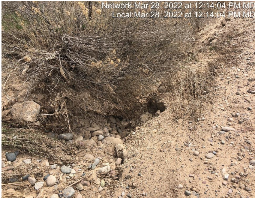
Photo #6316 Rill erosion occurring in ditch.
