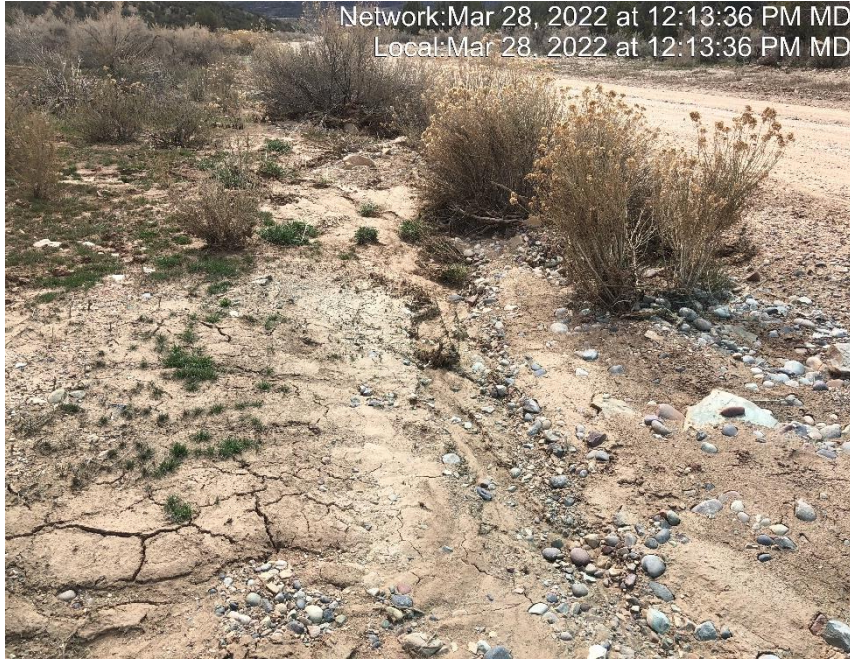
Photo #6314 Rill erosion occurring in ditch.
