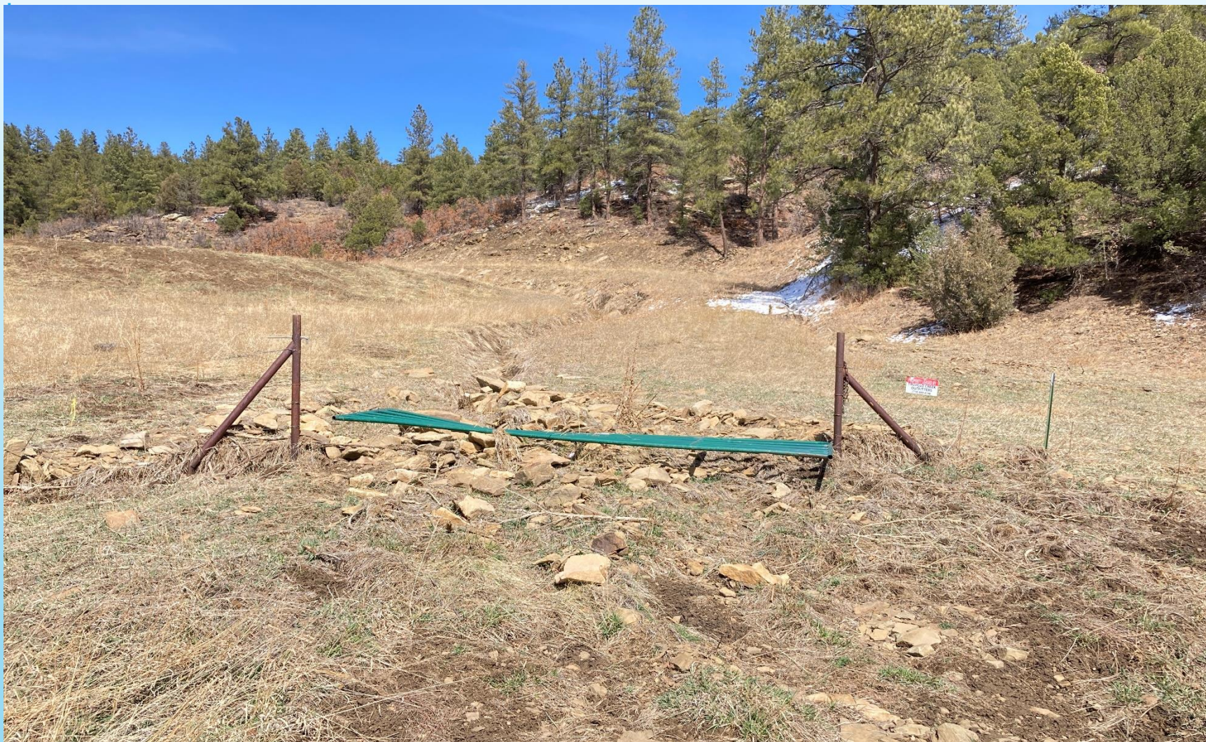
PHOTO 1: STORMWATER HAS WASHED OUT ROW AND KNOCKED DOWN THE GATE JUST OFF THE COUNTY ROAD. REPAIR GATE AND PROVIDE ACCESS TO LOCATION.
