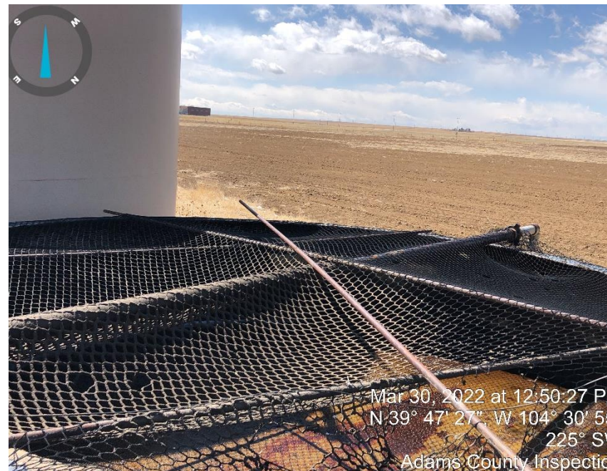
Photo #2 Open top tank (fluid in tank is less then 2 foot from the top).
