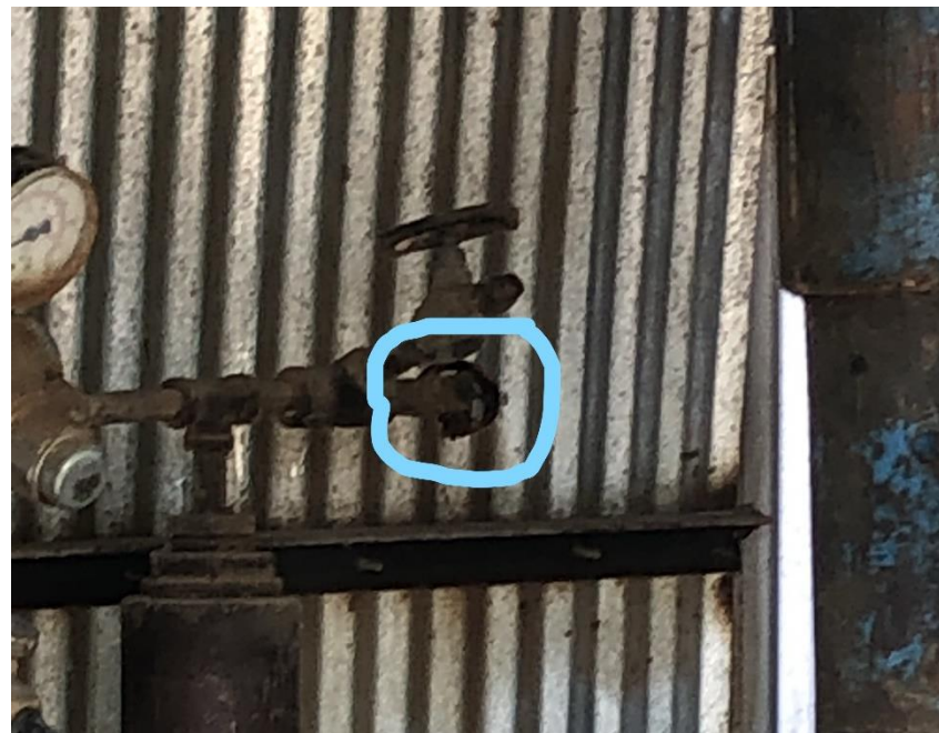
Photo #10 old valve leaking in well head house.
