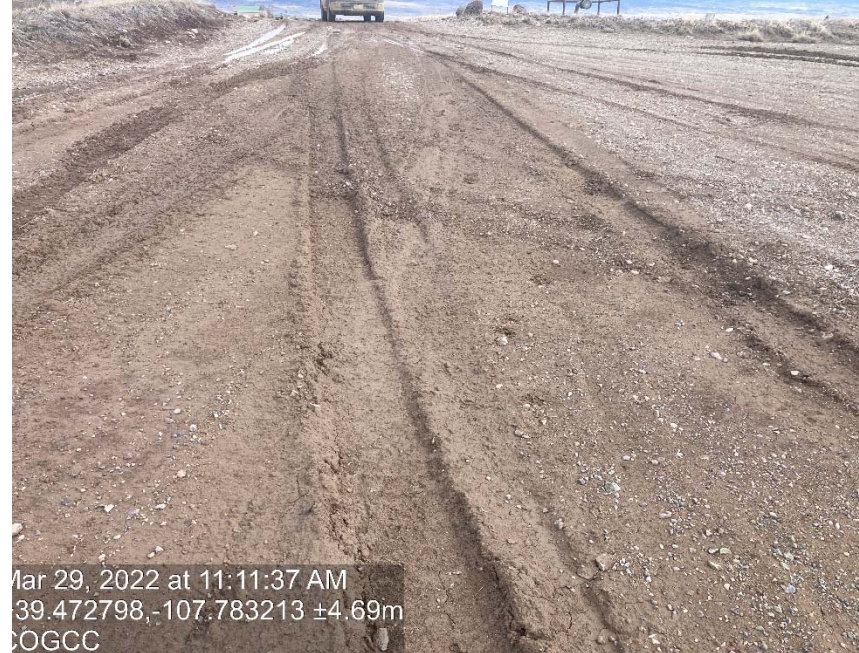
Lack of stabilization/compaction
