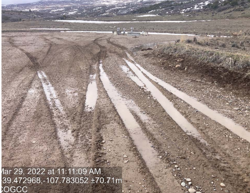
Lack of stabilization/compaction
