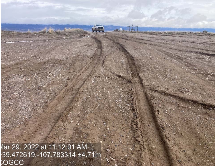
Lack of stabilization/compaction
