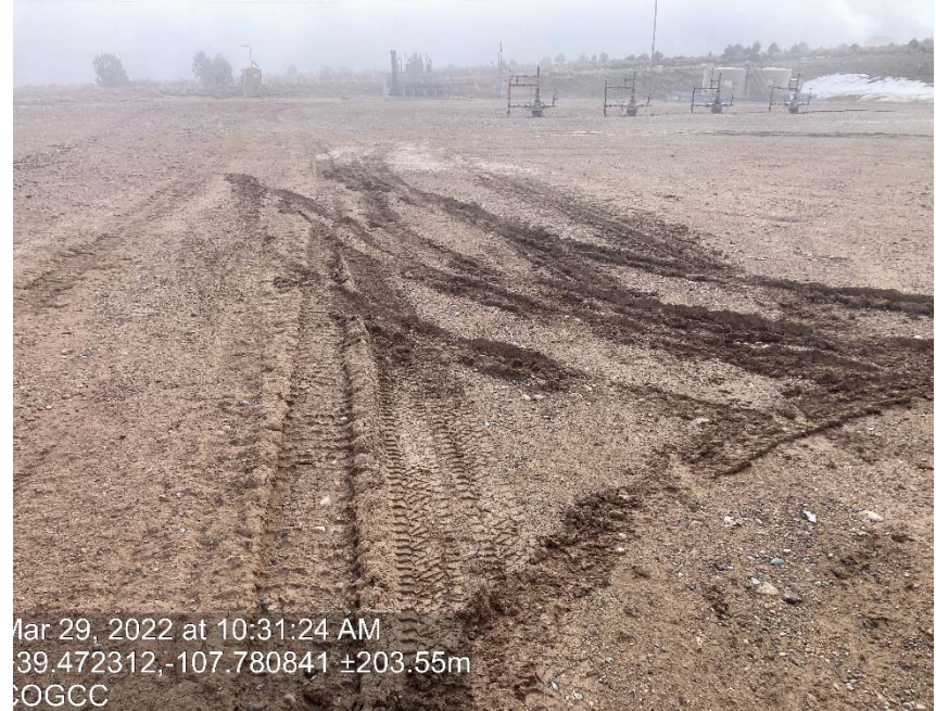
Lack of stabilization/compaction
