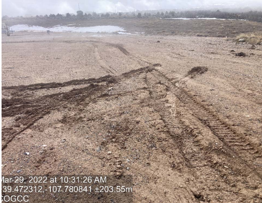
Lack of stabilization/compaction
