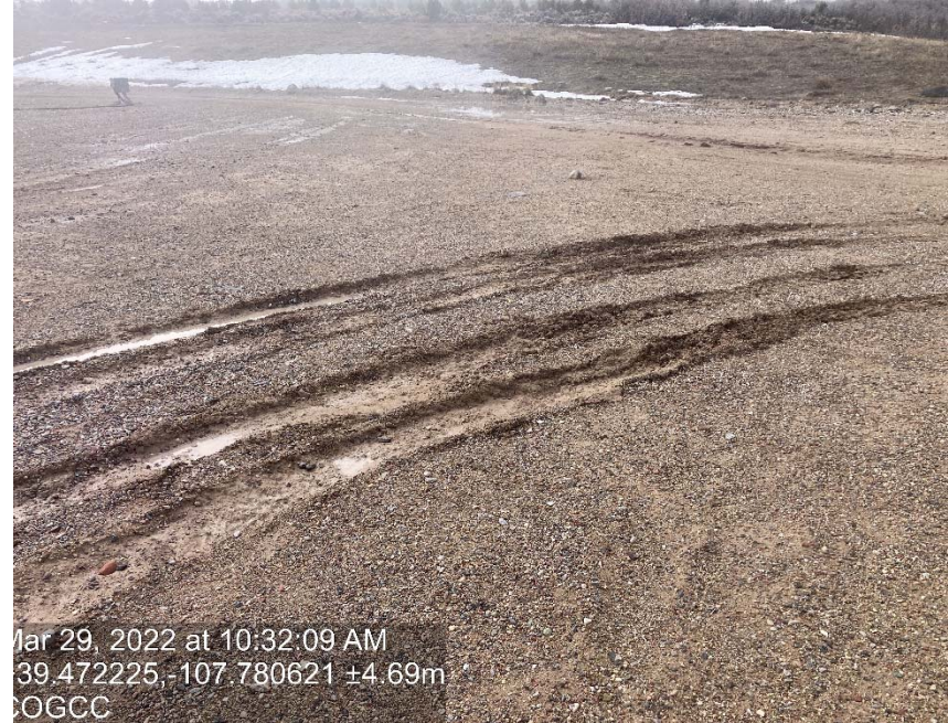
Lack of stabilization/compaction
