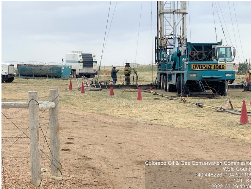
Photo #1 Printz 2-31 (05-123-13199) Wellsite Plugged & Abandoned | PA Plugging Operations: Kill well | WK Kill well, flaring gas
