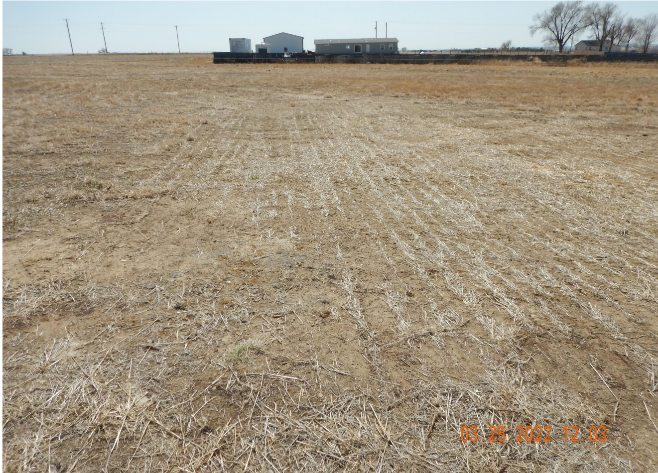
Photo 1. Photo taken from the well location, facing South. Photo illustrates Operator has performed final reclamation activities at the well location with the evidence of drill rows and straw crimped mulch. The well location has an open Remediation Project #17550.
