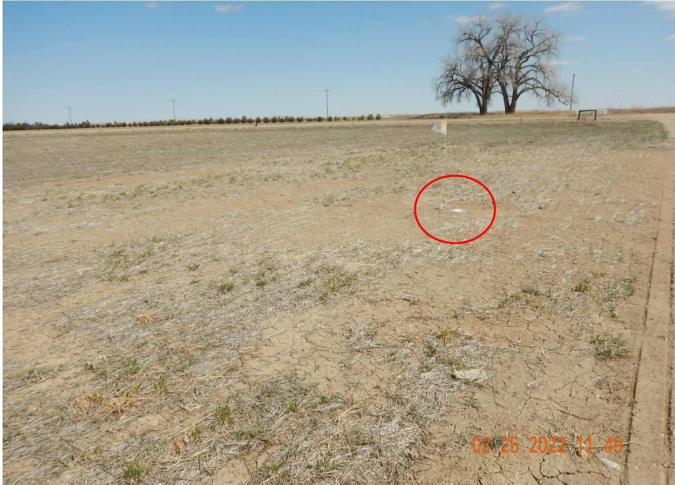
Photo 1. Photo taken from the well location, facing East. Photo illustrates Operator has performed final reclamation activities at the well location with the evidence of drill rows and straw crimped mulch. The well location has an open Remediation Project #17069. Photo illustrates one of the monitoring wells.
