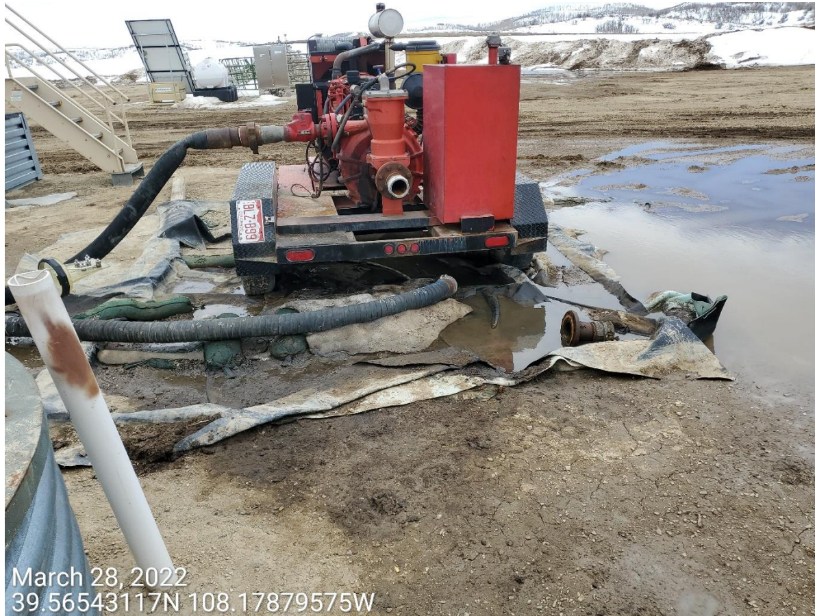
Photo 2: Photo of pump trailer and stormwater; liner/secondary containment BMP at pump inadequate to prevent spills and contamination of stormwater. Stained soils around pump equipment/liner evident.
