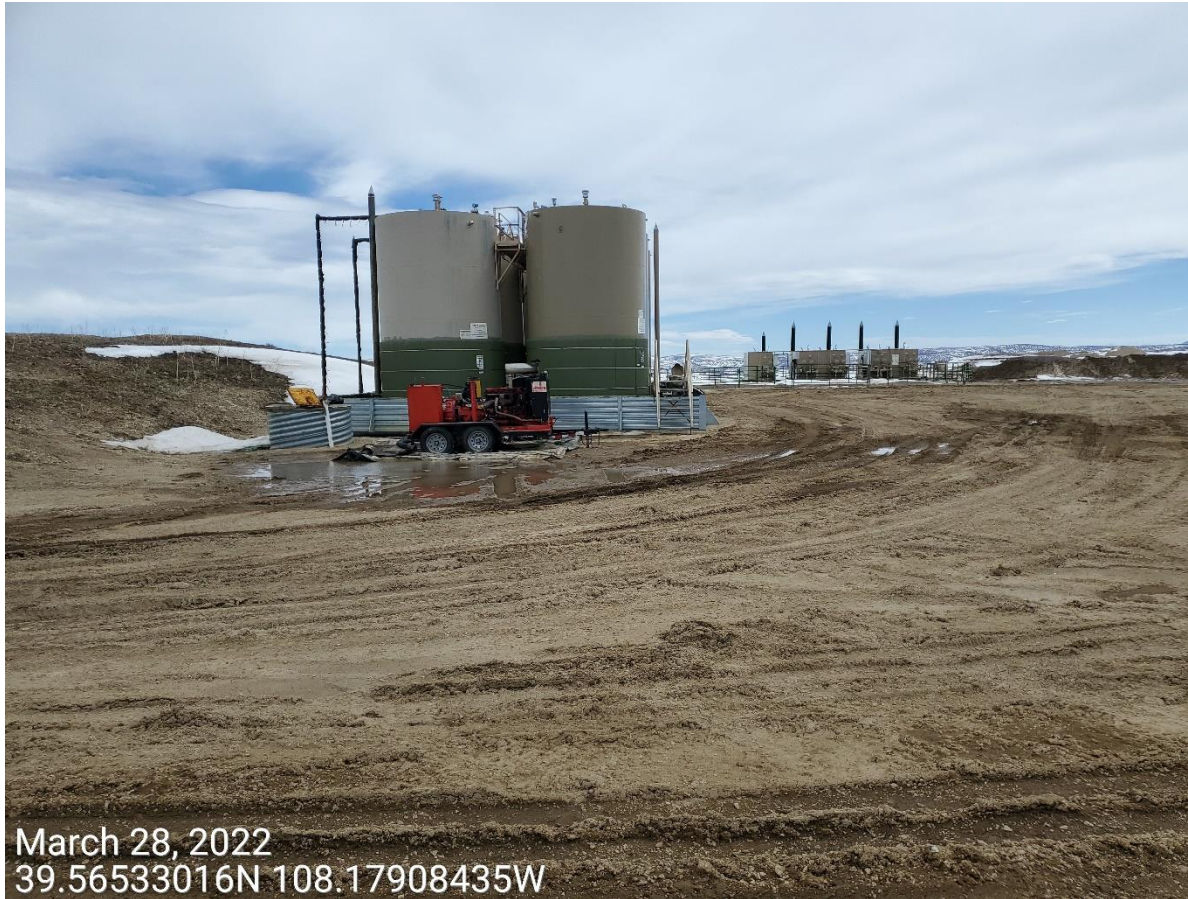
Photo 1: Photo shows pump trailer stored on the west end of the battery facility. Photo also shows stormwater ponding around equipment.
