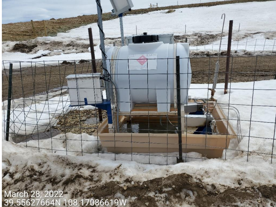
Photo 3: Photos show methanol tanks on the Location. BMPs to prevent wildlife access is missing from the secondary containment.
