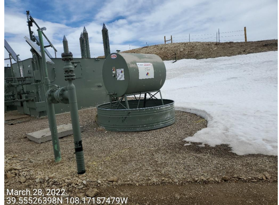
Photo 3: Photos show methanol tanks on the Location. BMPs to prevent wildlife access is missing from the secondary containment.
