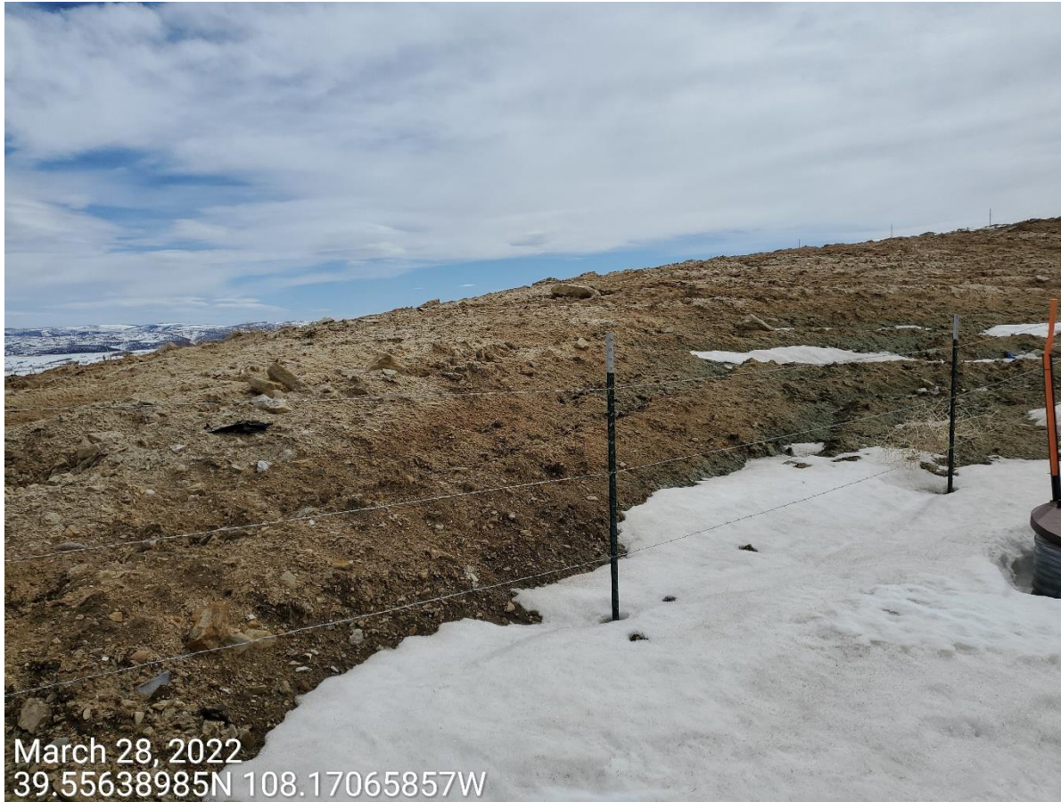
Photo 2: Interim areas of the Location; Areas appear to be hydroseeded and a soil binder implemented to stabilize the seeded soils
