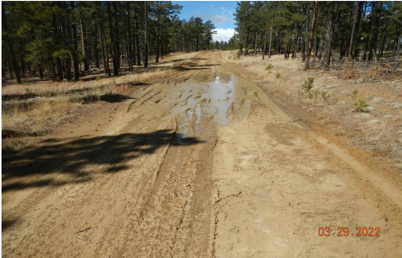
Photo 1. There is stormwater pooling on the road causing vehicle rutting and widening of the road. This area needs to be repaired and stabilized. Approx. Lat/Long:37.02629,-104.85264.
