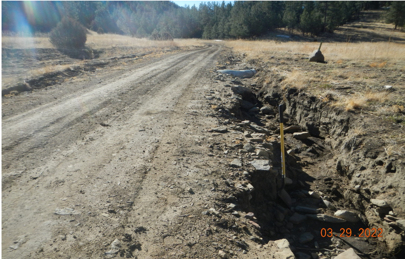
Photo 1. Facing southeast along the main road at the upper part of Lorencito Canyon. There is erosion along the road from recent storm event. Stormwater is bypassing the culvert. Previous corrective action was not completed.
