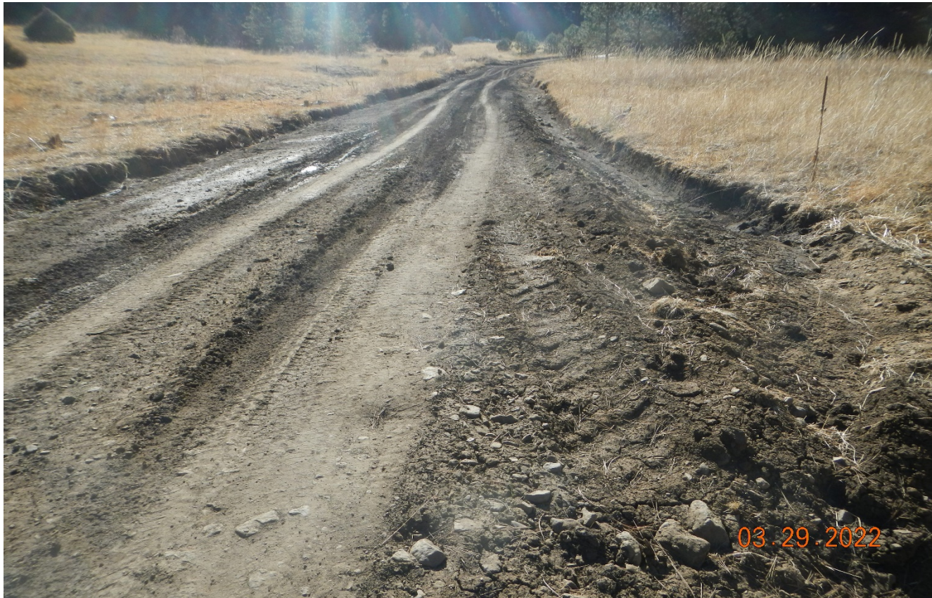
Photo 2. The culvert along the road is filled in with sediment causing stormwater to flow down the side of the road. Lat/Long:37.00499,-104.83742. Previous corrective action was not completed.
