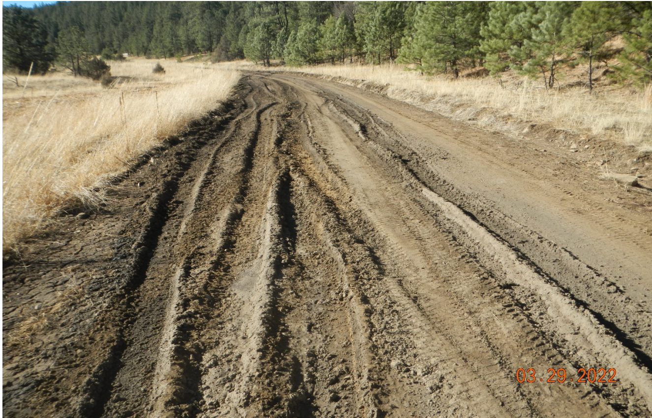
Photo 3. The road along the canyon is not stabilized and there is rutting and vehicle tracking occurring. The road needs to be repaired and stabilized.
