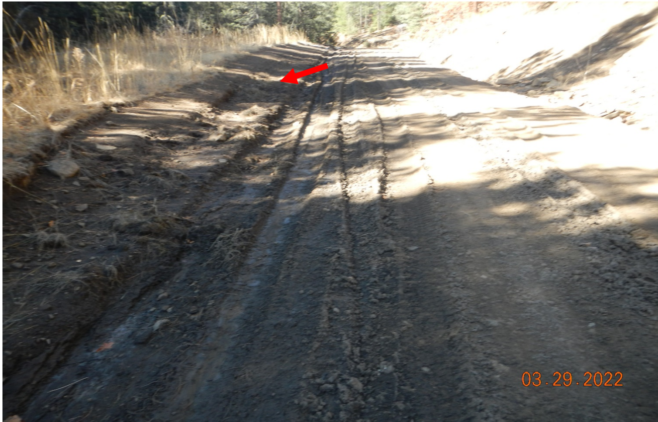
Photo 7. There was grading performed along the road. The disturbance along the side of the road shown at red arrow needs to be seeded and reclaimed. Previous corrective action not completed.
