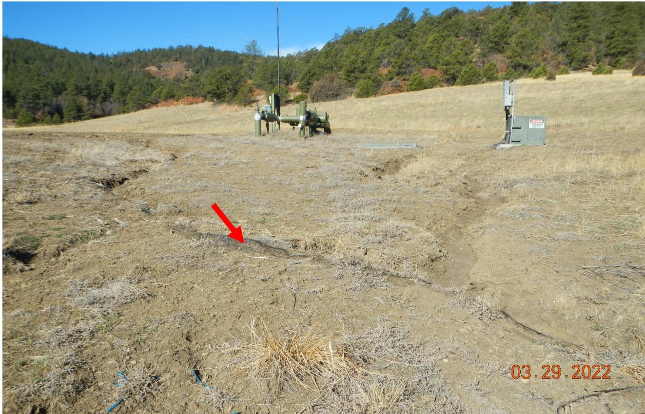
Photo 3. Facing toward the northeast side of the location. This area is not stabilized and there is an erosion. The wattles are degraded shown at red arrow. Previous corrective action not completed.
