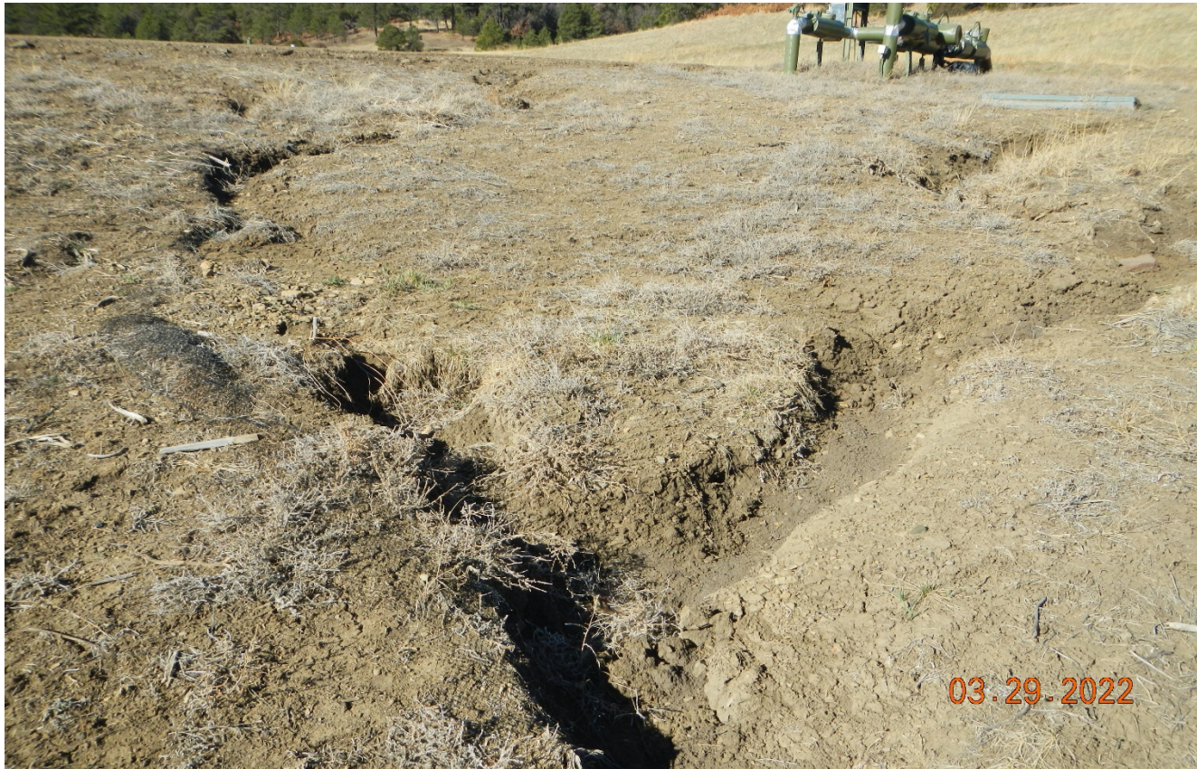
Photo 4. Facing toward the northeast side of the location. This area is not stabilized and there is an erosion channel that will need to be repaired. Previous corrective action not completed.
