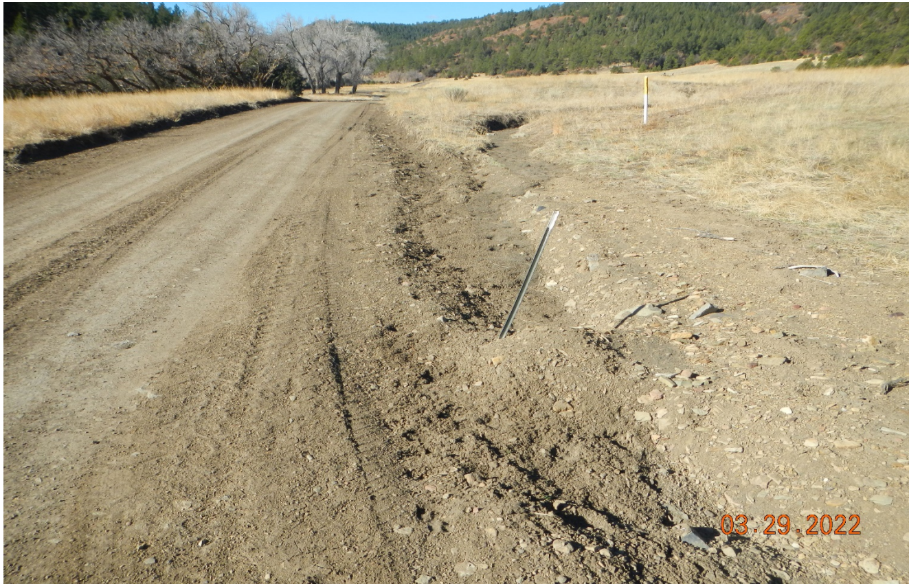
Photo 1. Facing southwest along the main road near the well site. Stormwater has washed across the road causing erosion. The culvert is filled in with sediment and has not been repaired. Previous corrective action not completed.
