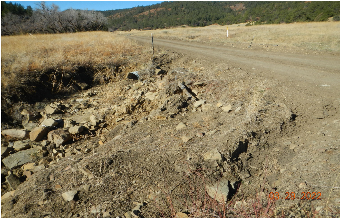
Photo 2. The culvert outlet is eroded and has not been repaired. No culvert outlet protection installed. Previous corrective action not completed.
