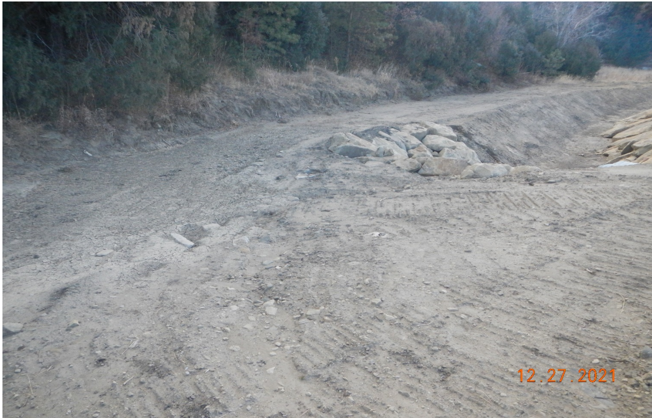
Photo 4. Facing at south side of the road at the additional culvert inlet. Disturbed bare soils have not been seeded and stabilized.
