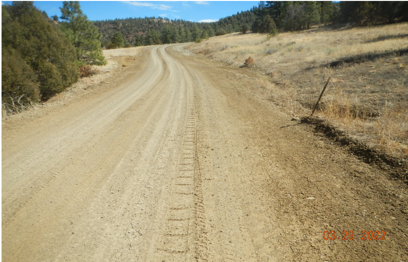
Photo 5. Facing northeast along the road. Areas of erosion along the road side have been filled in and repaired.
