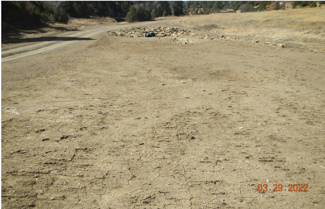
Photo 2. The disturbed bare soils along the roadside at the creek crossing have not been seeded and stabilized. Previous corrective action was not completed.
