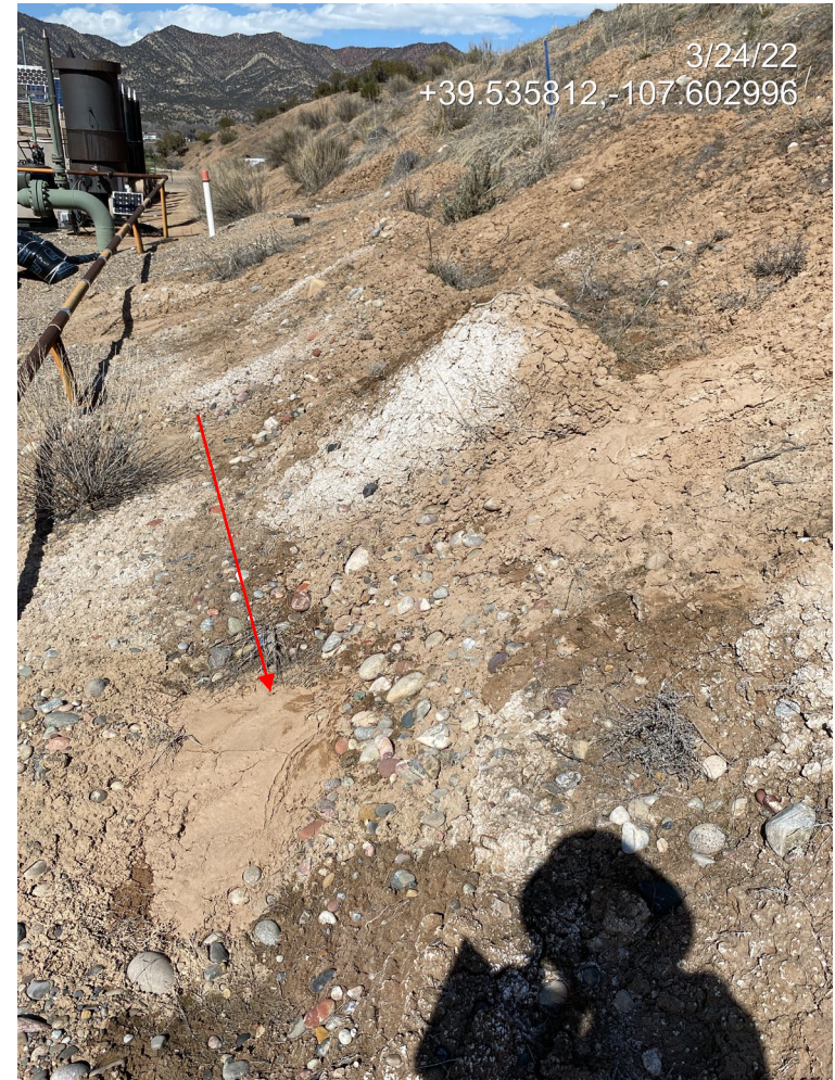
Photo 8. Photo taken from the eastern slopes of the Location shows sediment eroding and accumulating at the base of the cut slopes.
