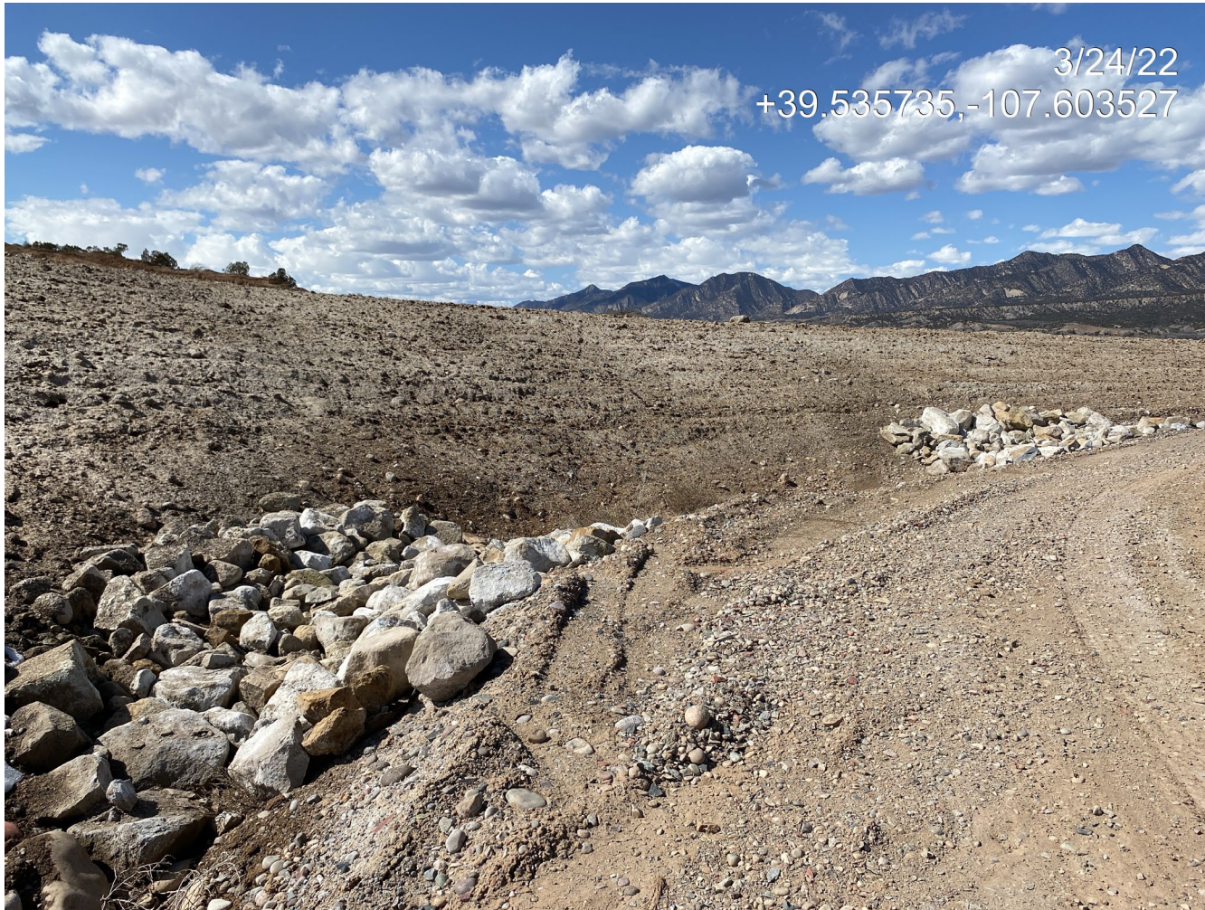
Photo 11. Photo taken from the southwest of the working pad area facing northwest shows a perimeter stormwater swale which was lined with geotextile fabric and angular rip-rap.
