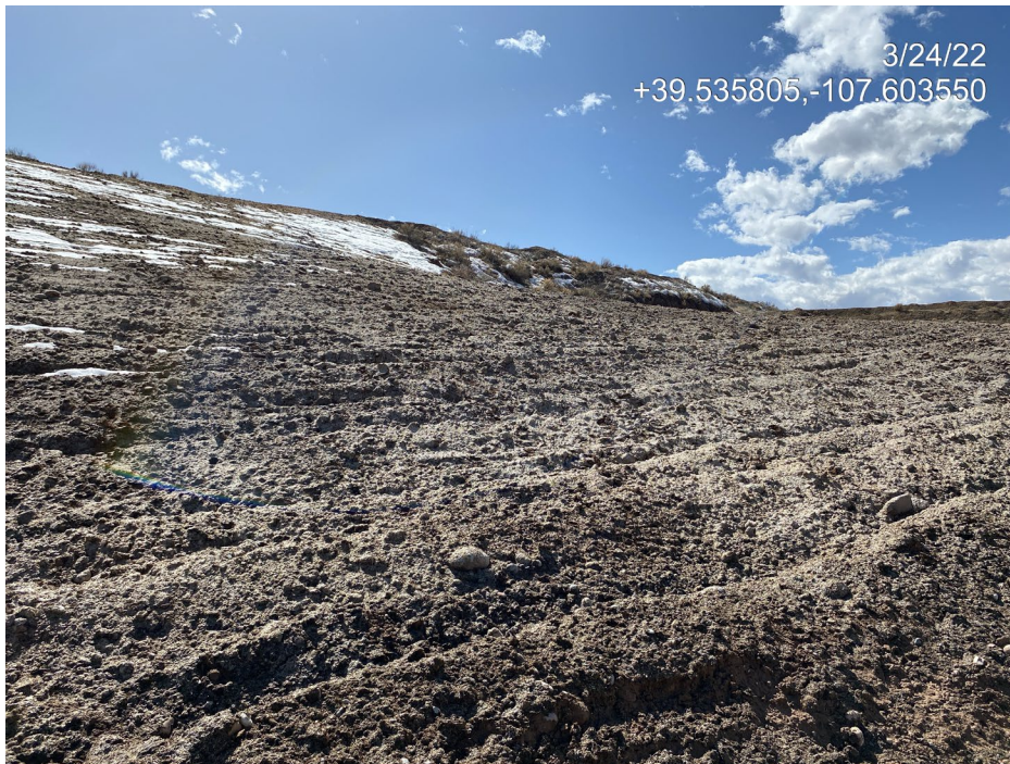
Photo 5. Photo taken from the southwest of the Location facing south shows interim area slopes have been hydromulched.
