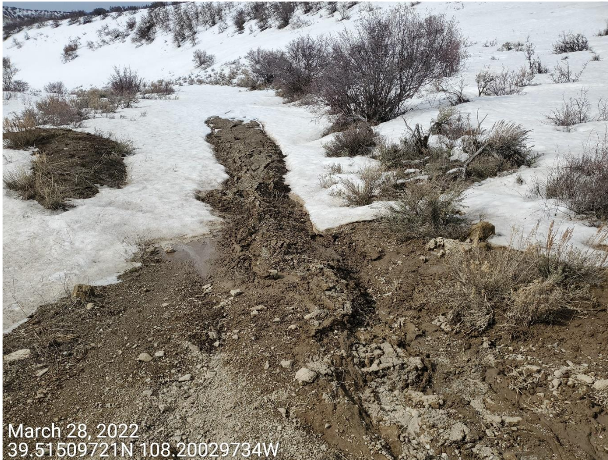
Photo 8: Photo shows sediment deposition due to erosion degradation and sediment transport from the access road.
