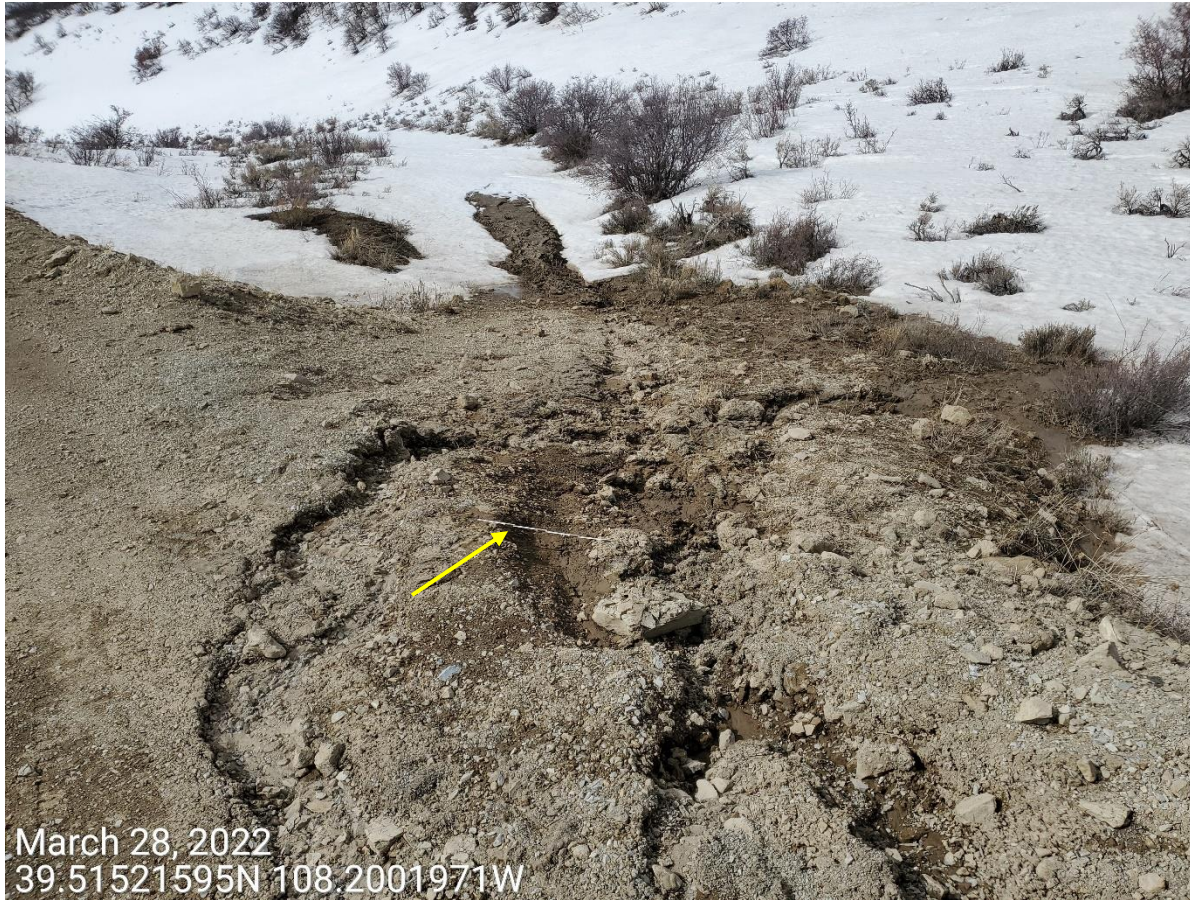
Photo 7: Photo taken from the access road on the north end of the Location. Photo shows erosion degradation has persisted along access road; control measures to stabilize, manage runoff and minimize erosion and sediment transport remains missing or insufficient at access road. 2 foot measuring stick for reference (arrow).
