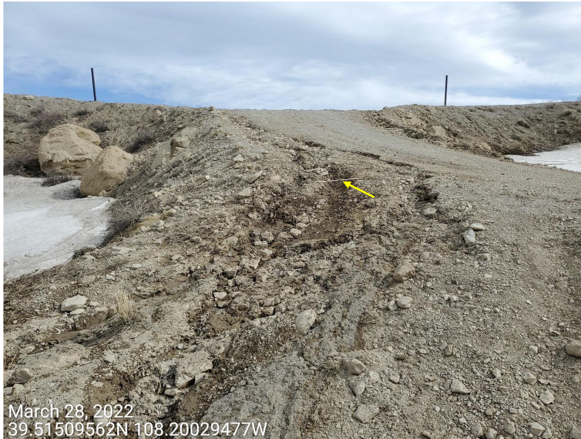
Photo 5: Photo taken from the access road on the north end of the Location. Photo shows erosion degradation has persisted along access road; control measures to stabilize, manage runoff and minimize erosion and sediment transport remains missing or insufficient at access road. 2 foot measuring stick for reference (arrow).
