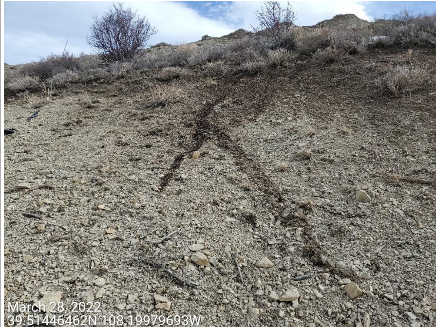
Photo 4: Photos taken from the slopes on the North/East end of the Location. Photo shows erosion and sediment transport.
