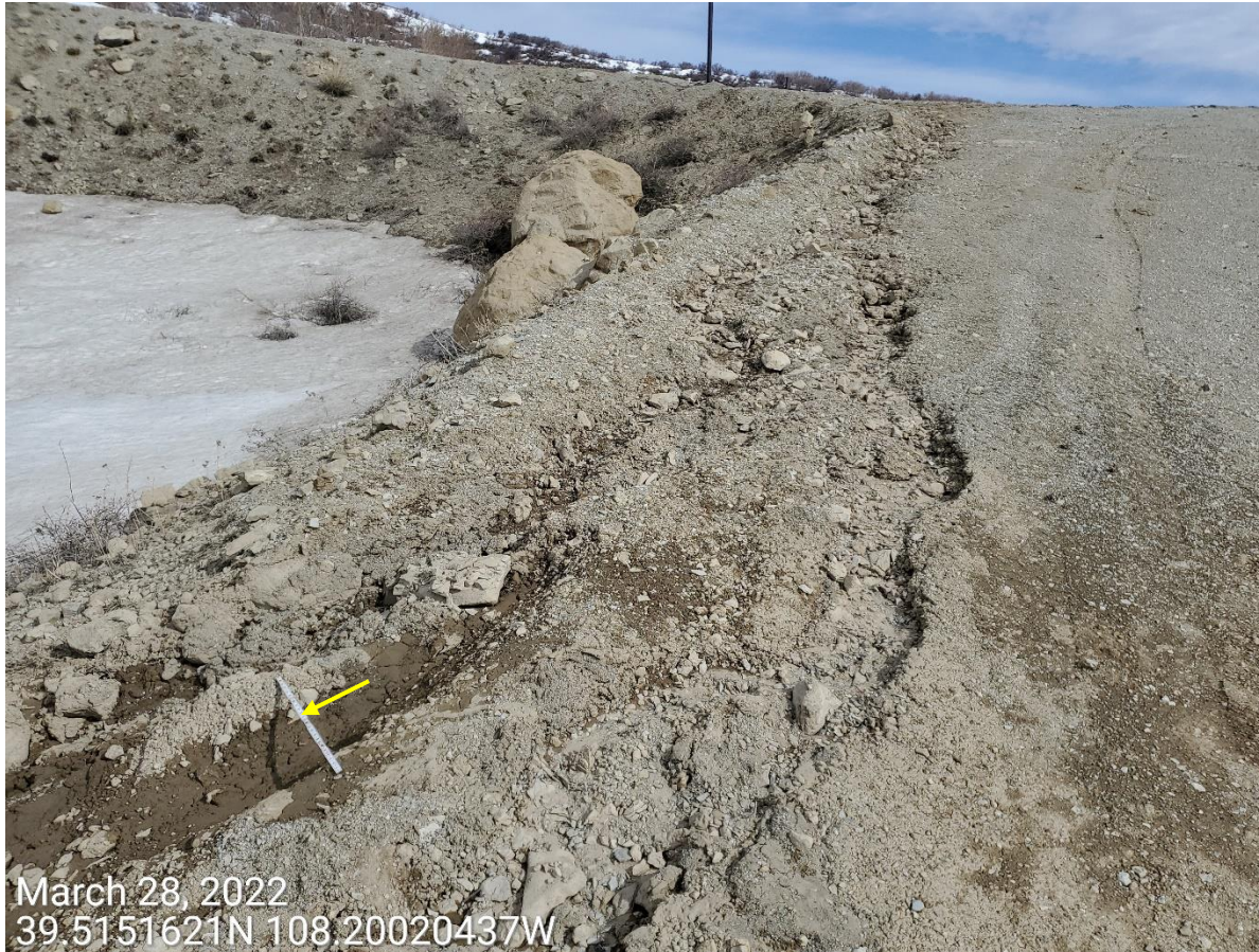
Photo 6: Photo taken from the access road on the north end of the Location. Photo shows erosion degradation has persisted along access road; control measures to stabilize, manage runoff and minimize erosion and sediment transport remains missing or insufficient at access road. 2 foot measuring stick for reference (arrow).
