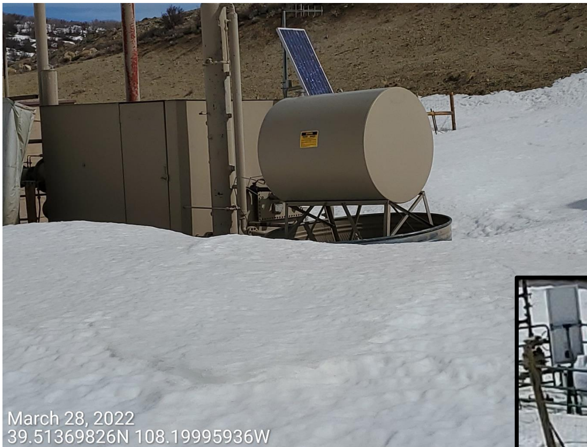
Photo 1: Photo shows wildlife protection devices to prevent wildlife access remain missing or insufficient from the secondary containment BMPs at the tanks.
