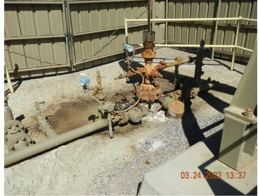
Stained and wet area around #17-3 well head.
