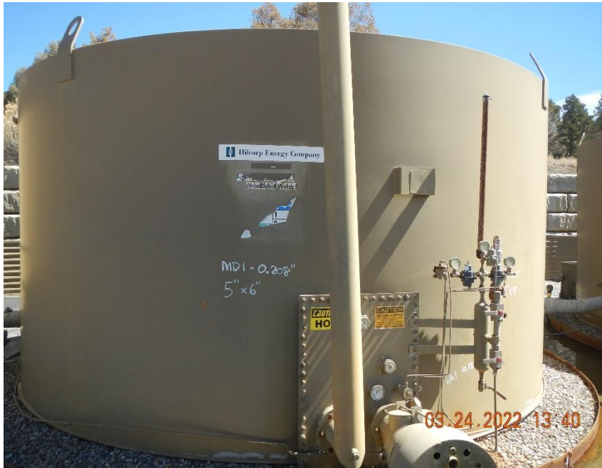
Illegible labels on northern AST.
