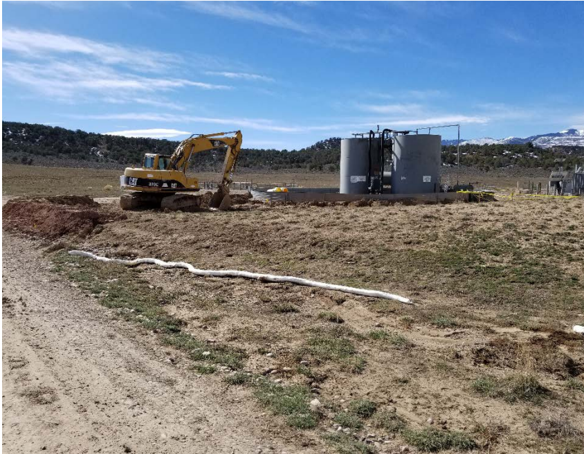
Photo #5 – Overview of tank battery from north. Note excavator remaining in excavation area and installation of absorbent boom downhill from excavation.
