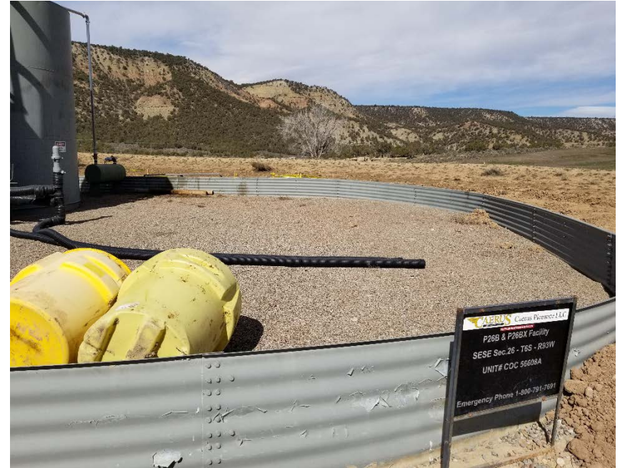
Photo #12 – North end of tank battery, looking west. Note no tank battery liner was observed on inspection date.
