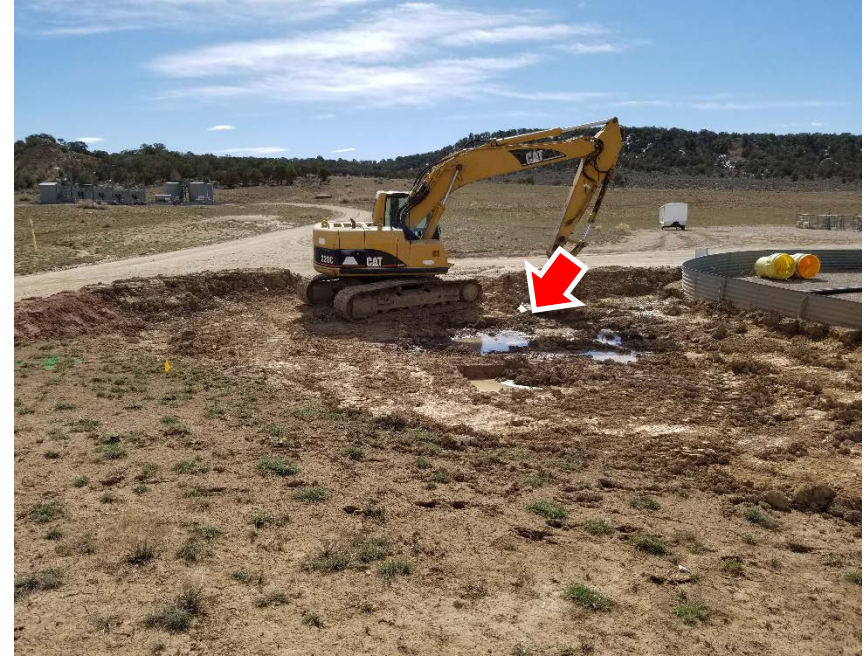
Photo #16 – View of north end of excavation. Note unidentified fluids remaining in tank battery (red arrow).
