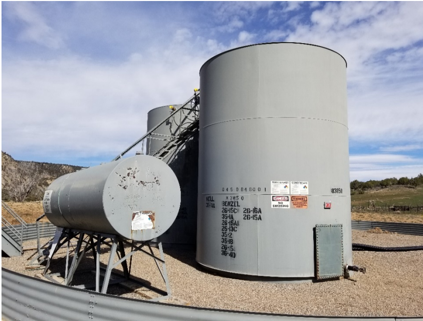
Photo #13 – Tank battery secondary containment ring contained two 300 bbl steel ASTs labeled to contain produced water and condensate and one 1000 gallon methanol tank on inspection date.
