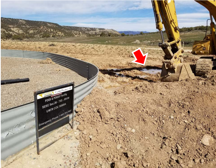
Photo #11 –View of excavation area north of tank battery. Note unidentified fluids were observed in this location on inspection date (red arrow).
