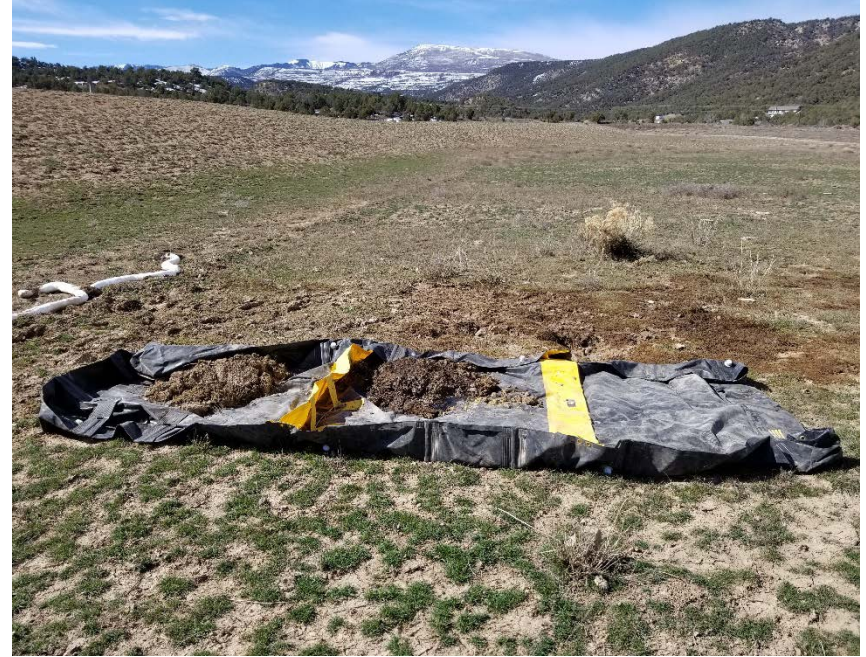
Photo #8 – Impacted soil stockpiled on liner in flow path area.
