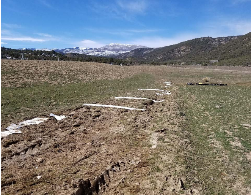
Photo #7 – Absorbent pads and booms installed by operator along flow path.
