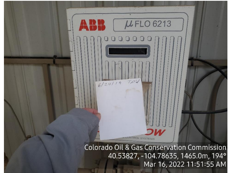
Photo 6: Meter not annually calibrated
