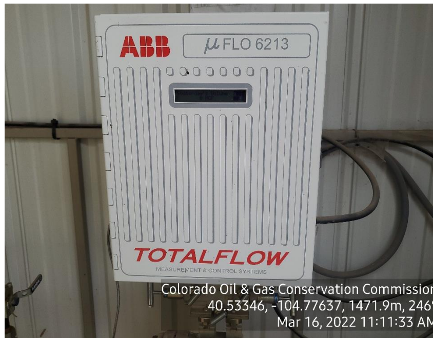
Photo 5: No calibration card displayed
