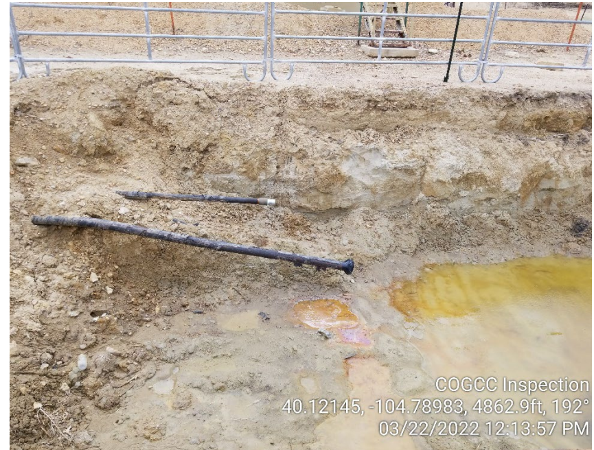
Photo 4 – Open excavation for Spill 480738. Groundwater with hydrocarbon sheen visible in excavation.
