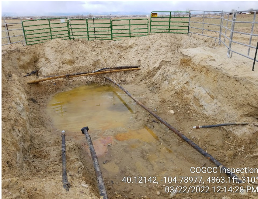
Photo 3 – Open excavation for Spill 480738. Groundwater with hydrocarbon sheen visible in excavation.
