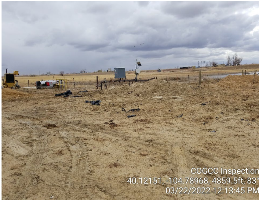
Photo 5 – Soils stored on location. Lining is torn and stormwater BMPs are inadequate.
