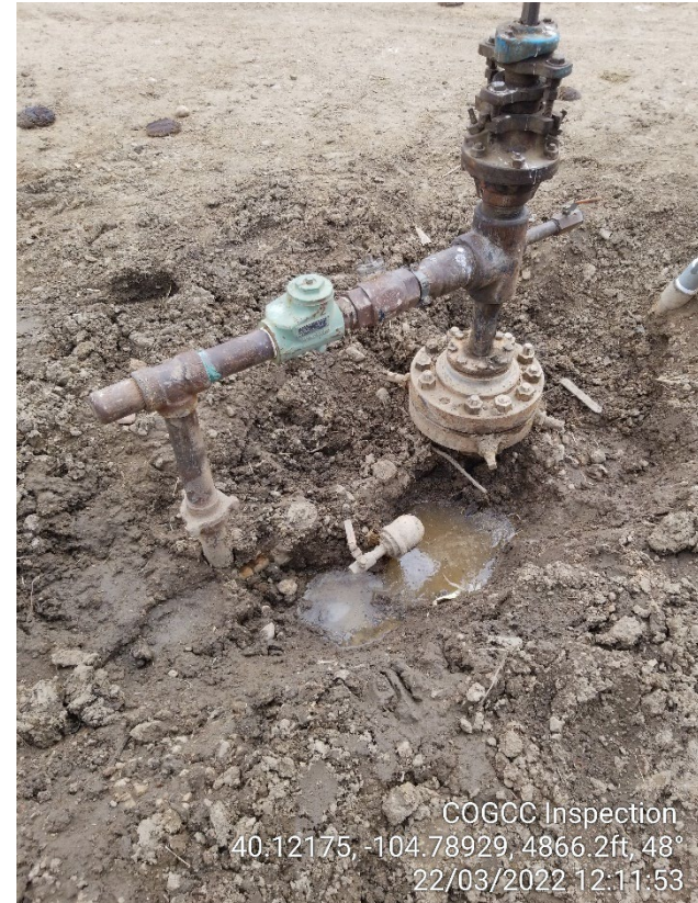
Photo 6 – Soils dug out around wellhead.
