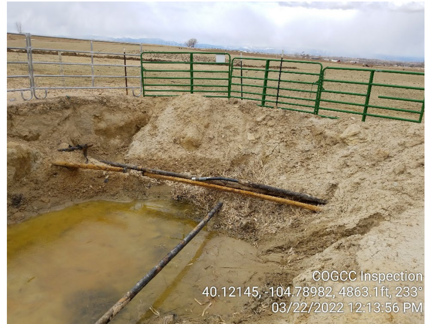
Photo 2 – Open excavation for Spill 480738. Groundwater with hydrocarbon sheen visible in excavation.
