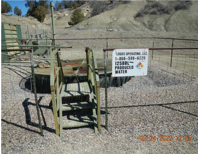
Carr #1M open topped PBV.
