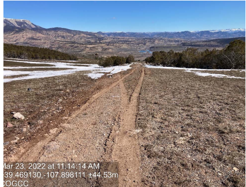
Lack of stabilization/compaction
