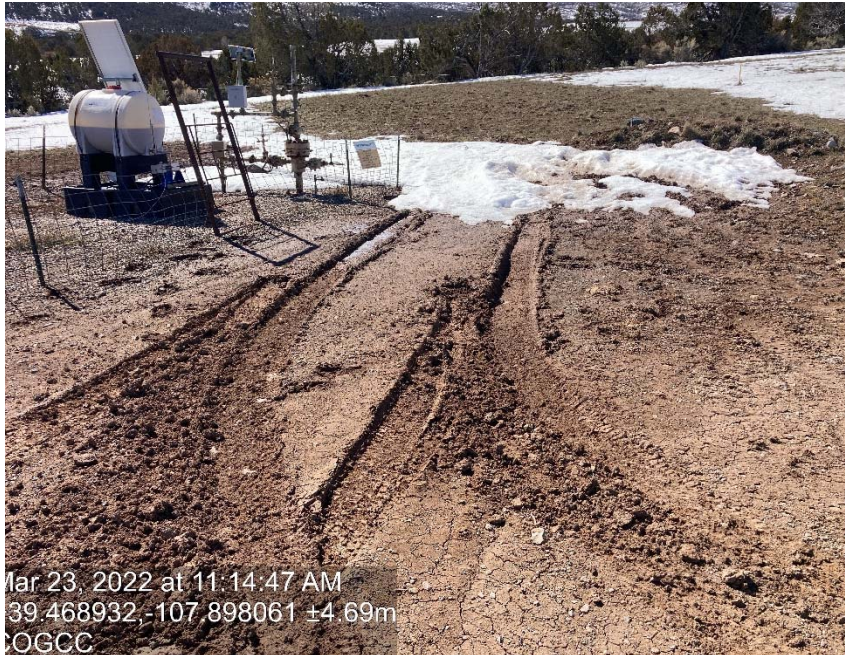
Lack of stabilization/compaction
