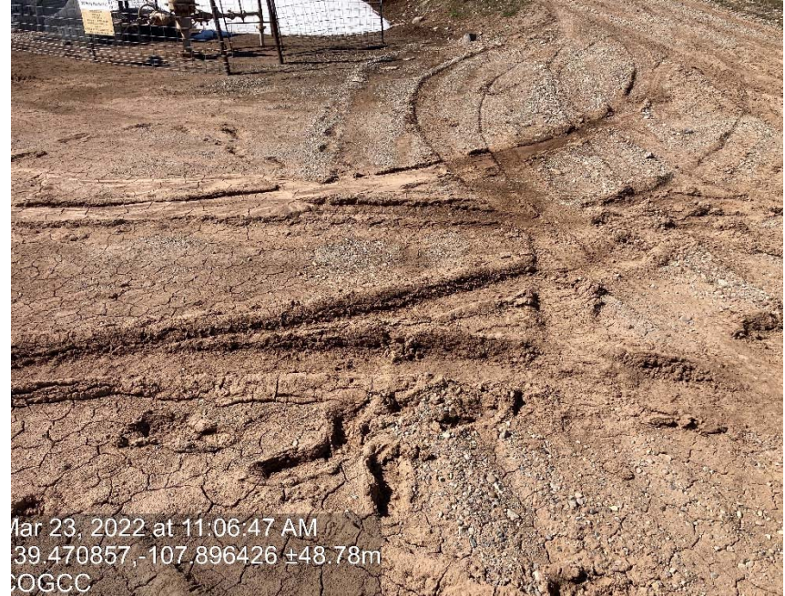
Lack of stabilization/compaction
