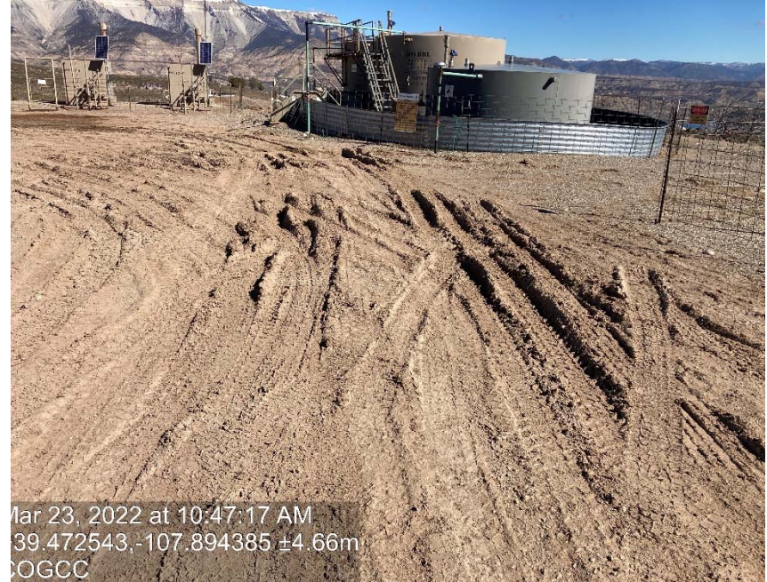
Lack of stabilization/compaction
