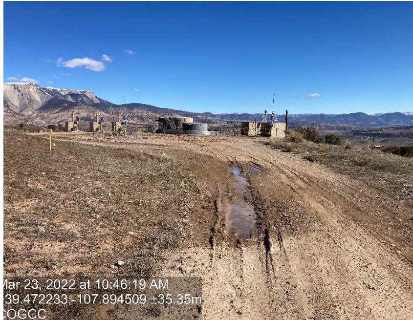
Location and Lack of stabilization/compaction
