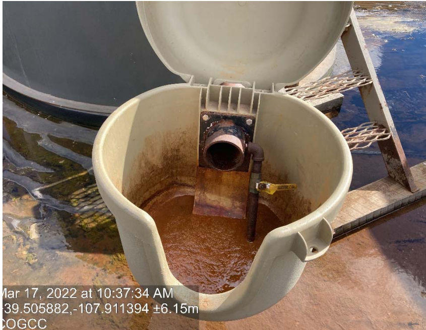
Valve missing cap/plug
