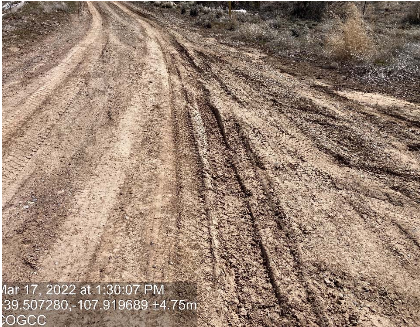
Lack of stabilization/compaction
