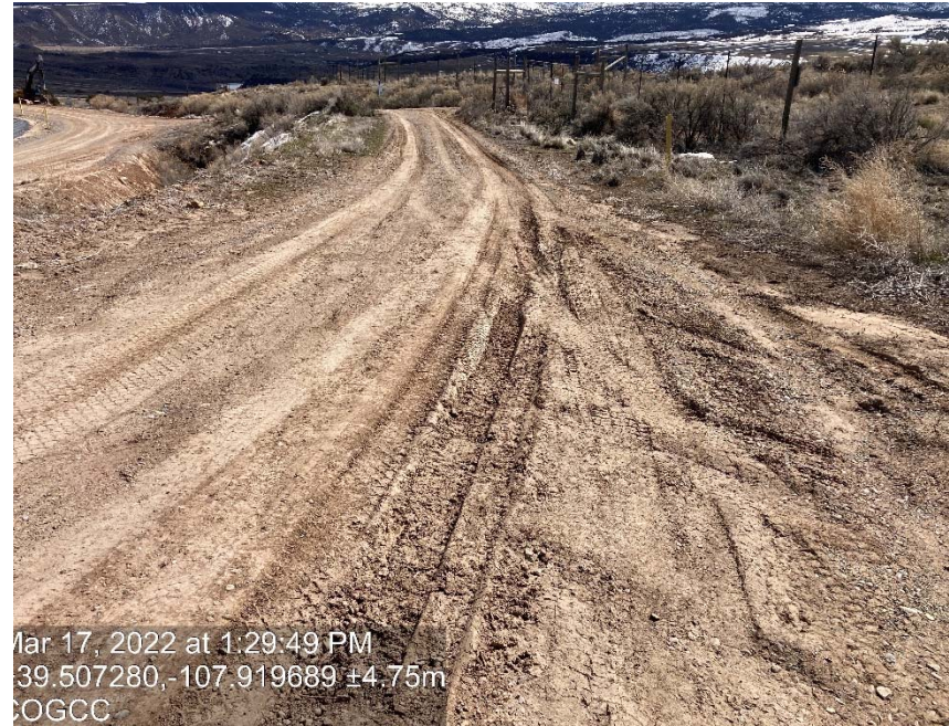
Lack of stabilization/compaction
