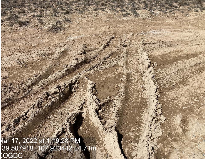
Lack of stabilization/compaction
