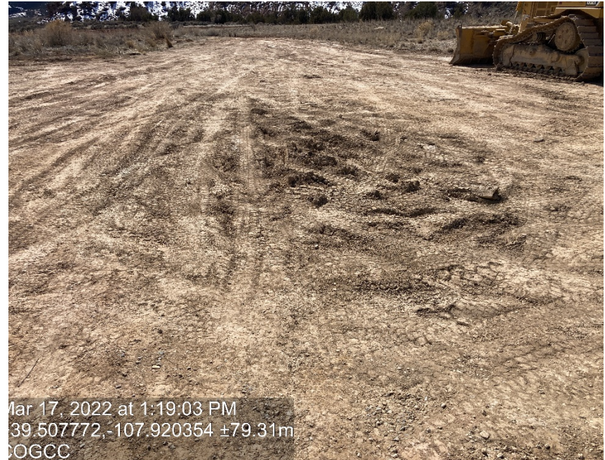
Lack of stabilization/compaction
