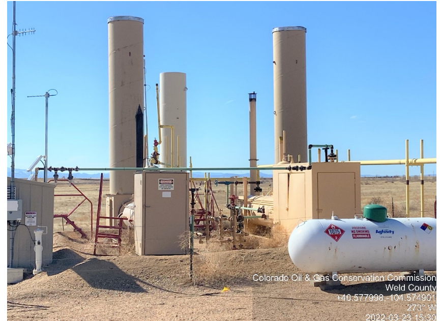
Photo #4 Kohlhoff USX AB 17-03P, 17-04P, 17-03P Battery site Active Separators, ECDs
