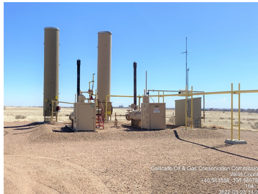
Photo #4 Waugh PC AB08-13 Battery site Active Separators, ECDs
