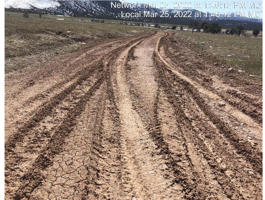
Photo #6311 Insufficient tracking control at entrance to location.
