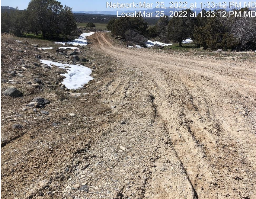
Photo #6307 Insufficient tracking control at entrance to location.
