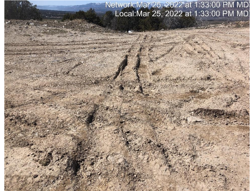
Photo #6306 Location lacks stabilization.
