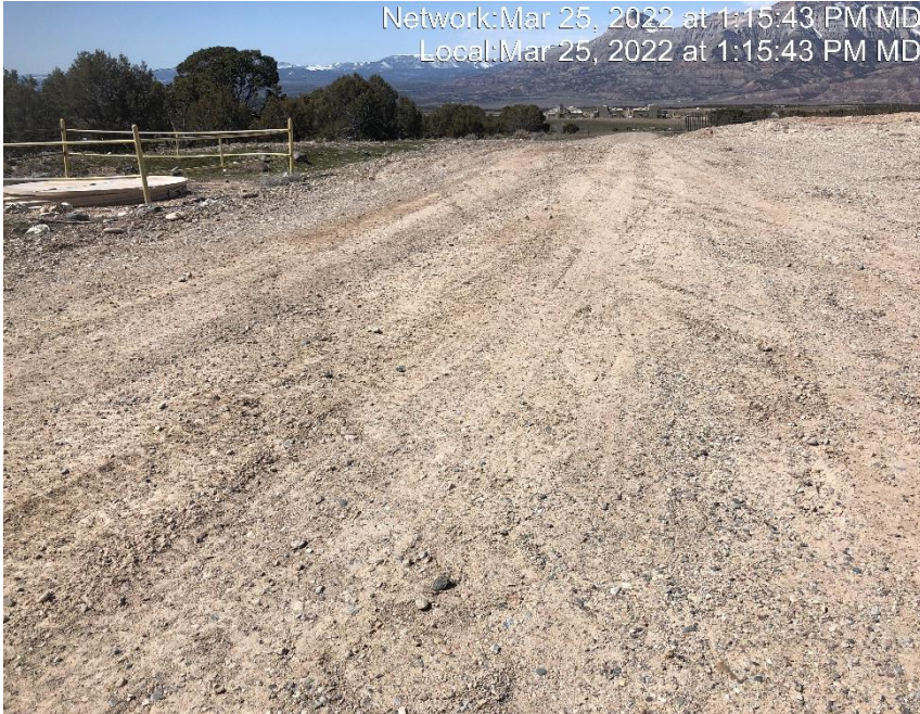
Photo #6302 Insufficient tracking control at entrance to location.
